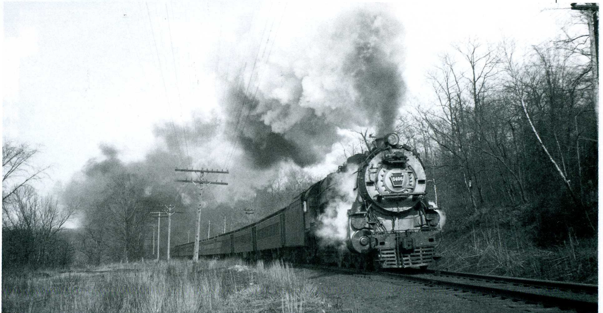
The earliest known photo of 5406 on LIRR, July 21, 1934, location Mineola, leading Train 12, Shinnecock Express . It's pretty much as delivered by Baldwin, and wearing the elegant LIRR trademark smokebox paint scheme. The large headlight, bar pilot and four-legged classification lights make this the most admired K4s design. (Charles B. Chaney photo; Ron Zinn collection)
