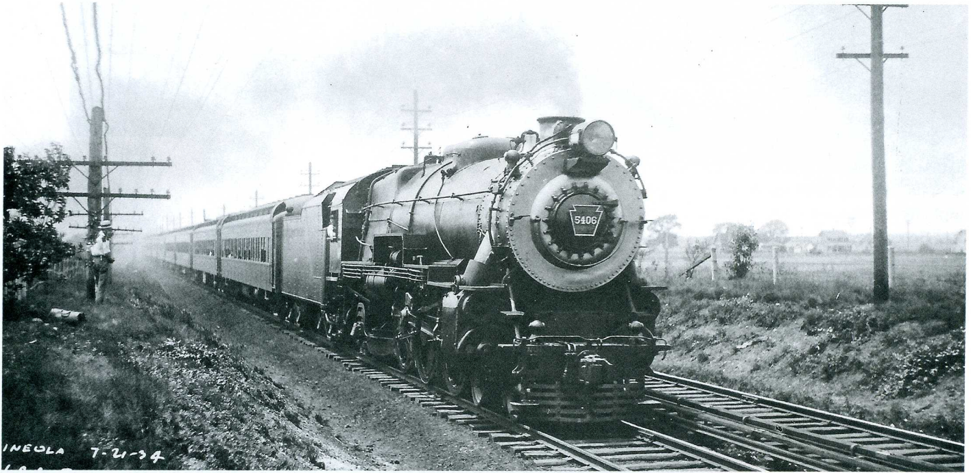
The earliest known photo of 5406 on LIRR, July 21, 1934, location Mineola, leading Train 12, Shinnecock Express . It's pretty much as delivered by Baldwin, and wearing the elegant LIRR trademark smokebox paint scheme. The large headlight, bar pilot and four-legged classification lights make this the most admired K4s design. (Charles B. Chaney photo; Ron Zinn collection)
