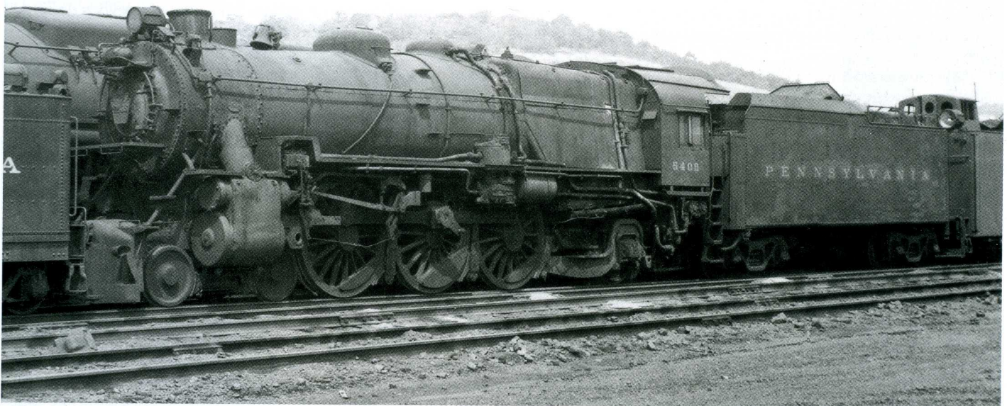
5406 was retired at East Altoona in August 1957. Its drive rods in the tender, it awaits disposition among J1's, H10s's, and other K4s's. Its bell, headlight, keystone, and perhaps badge plates will be removed before being sold as scrap in February 1958. Note the web-spoked main driver. (Author's collection)
