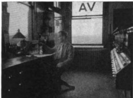
Operator's table at Valley Stream, showing concentration unit on table and the telephone and telegraph test panel in the background
