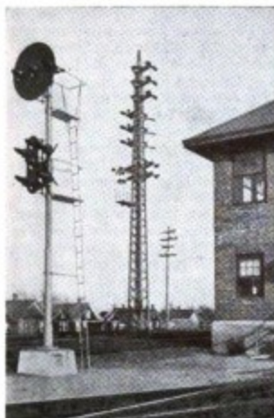
Steel lattice junction pole opposite high-tension rack at tower
