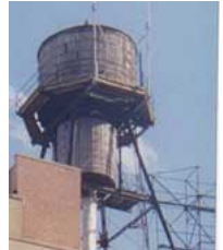
Water Tank, American Stove Company, Spot 14 Credit: Bill Myers
