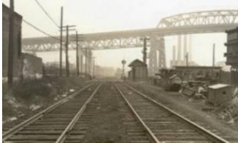
Shaw Walker (Spot 10) on left, Penny Bridge Shed in background on right side of track. Jacobson would be on left. Camera looking East. Kosciusko Bridge, which replaced Penny Bridge in the 1930s, in the background. Official LIRR photographer, probably Weber 1940. Credit: Collection of Art Huneke
