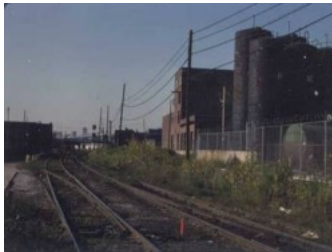
Stoll Metal (Spot 2) was on the right hand side of the tracks beyond Van Iderstine Spots 5a and 5b (beyond the vertical tanks) at right side of photograph (photo looking West). Spot 5c is on left side of photograph, past switch. Greenpoint Avenue Bridge in background. Vantage point is furthest East of all photos appearing in this article. Arthur Huneke, September 10, 1982, Color Slide, Credit: Arthur Huneke Collection
