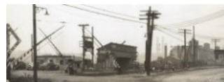
Laurel Hill Boulevard Crossing Building on the right background with two towers is Marlyn Warehouse (Spot 7) Camera looking North West LIRR Photograph Circa 1940. Credit: Art Huneke
