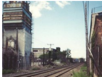
Leftmost structure is a cement silo operated by Princepe-Dana. Building on the center left background is Marlyn Warehouse (Spot 7) Camera looking Northwest Carl Fabrizio 1998. Credit: Carl Fabrizio
