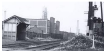
2 Marlyn Warehouse (Spot 7) Note twin prominent elevator or staircase shafts. Penny Bridge Station Shed at left foreground. Note absence of cement silo. William D. Slade July 1953. Credit: Art Huneke Collection
