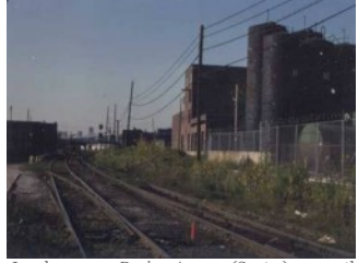
Centre Lumber, 37-10 Review Avenue (Spot 3) was on the right hand side of the tracks beyond Van Iderstine Spots 5a and 5b (beyond the vertical tanks) at right side of photograph (photo looking West). Spot 5c is on left side of photograph, past switch. Greenpoint Avenue Bridge in background. Vantage point is furthest East of all photos appearing in this article. Arthur Huneke, September 10, 1982, Color Slide, Credit: Arthur Huneke Collection
