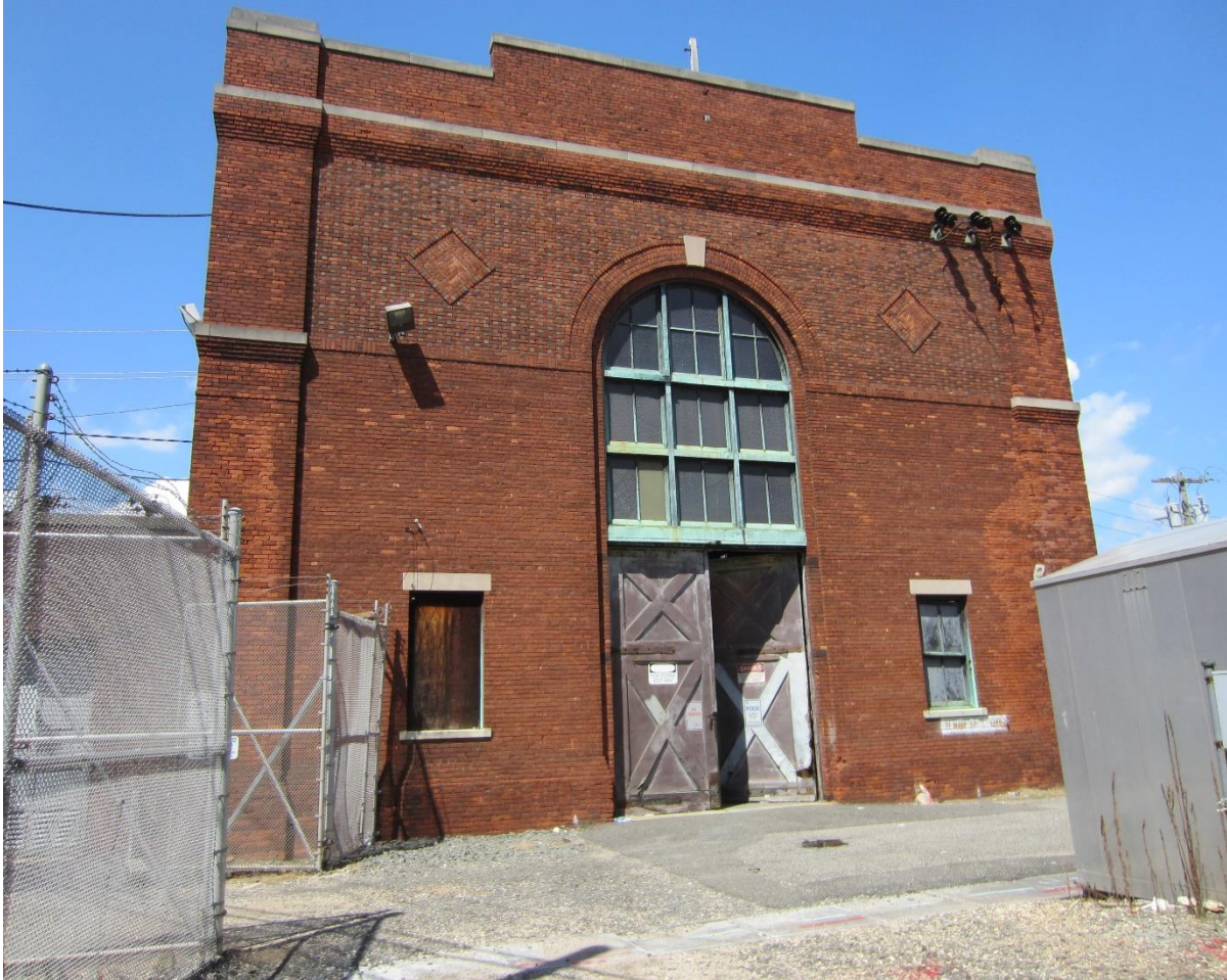
PHOTO 08. SOUTH ELEVATION OVERALL
