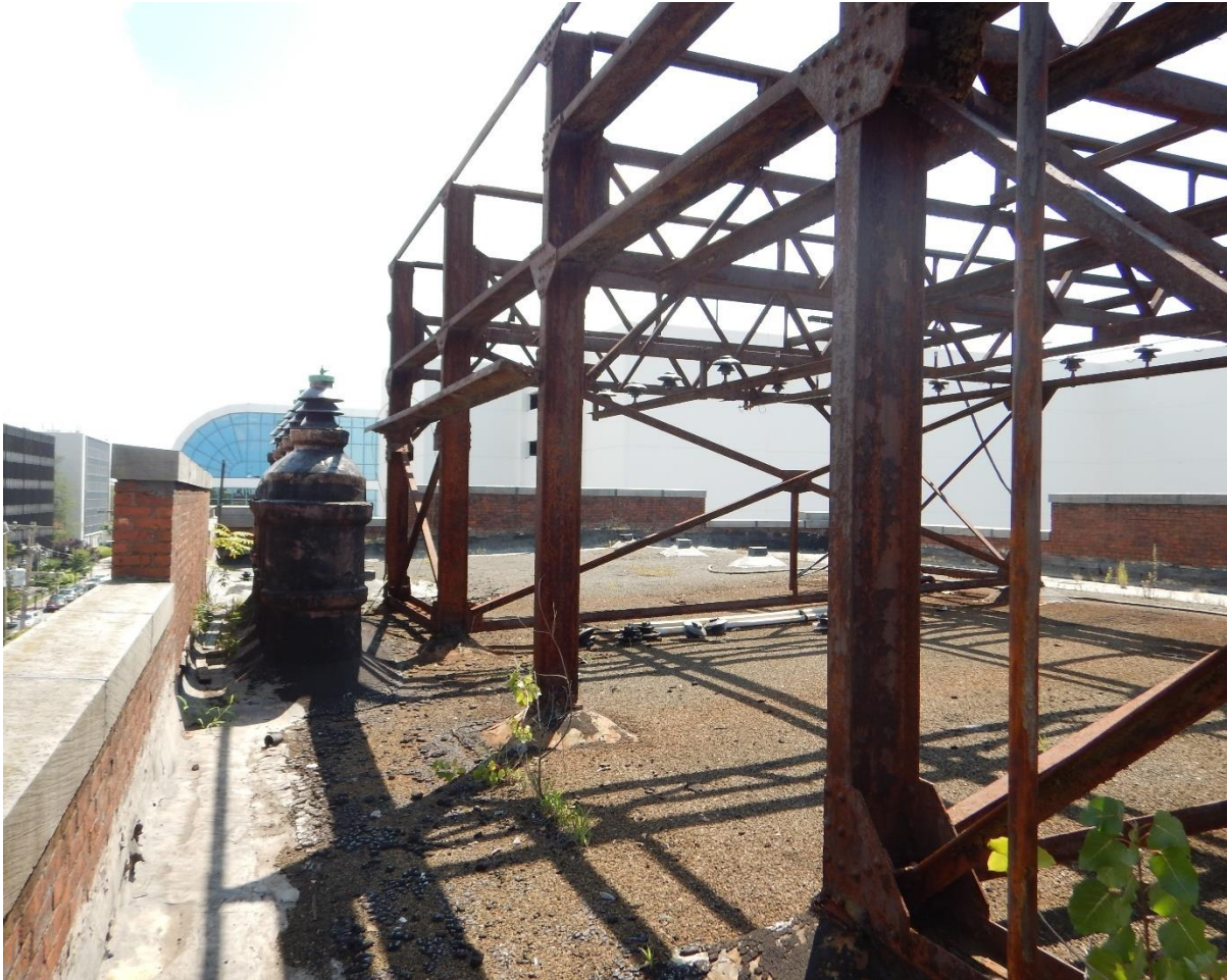
PHOTO 15. MAIN ROOF FACING SOUTH
