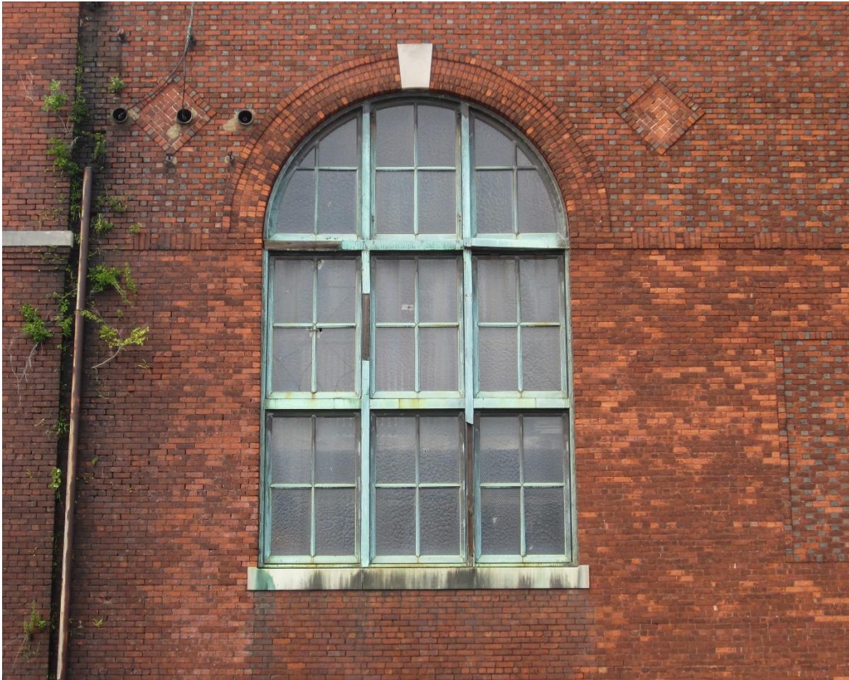
PHOTO 03. EAST ELEVATION WINDOW DETAIL
