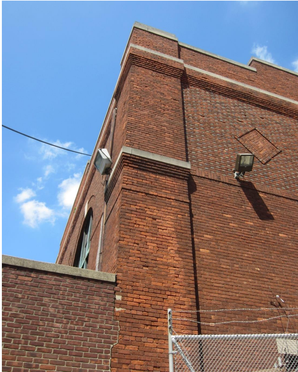
PHOTO 11. SOUTH ELEVATION BRICK DETAIL
