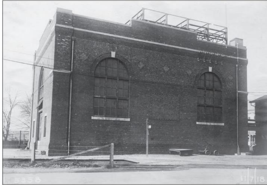
Fig. 7. The east and south facades of the Mineola Electrical Substation (substation No. 8) in a photograph dated November 7, 1918, eight years after the building's completion. View looking west from Main Street. The bridge between the substation and signal tower is still intact (visible at the far right). The garage addition has not yet been built. Little else had been altered between this photograph and the current appearance. Source: Long Island Rail Road: Oyster Bay Branch , 29.
