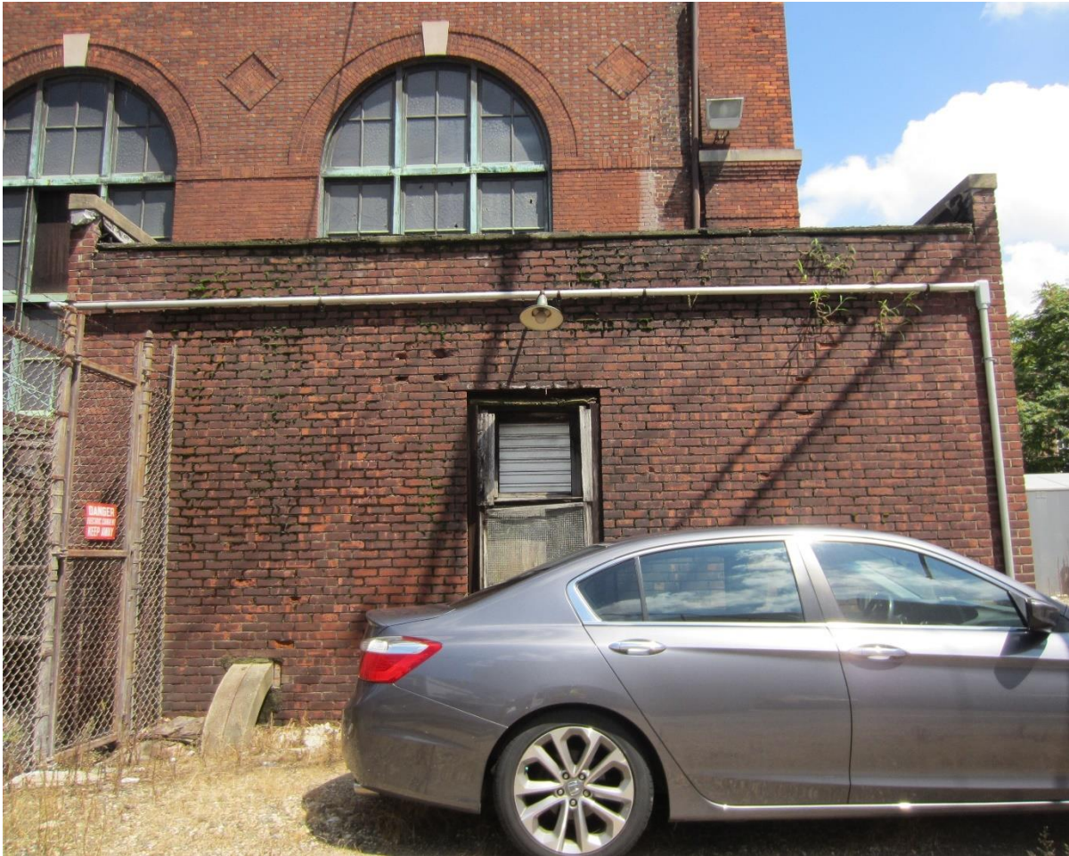
PHOTO 14. WEST ELEVATION ADDITION
