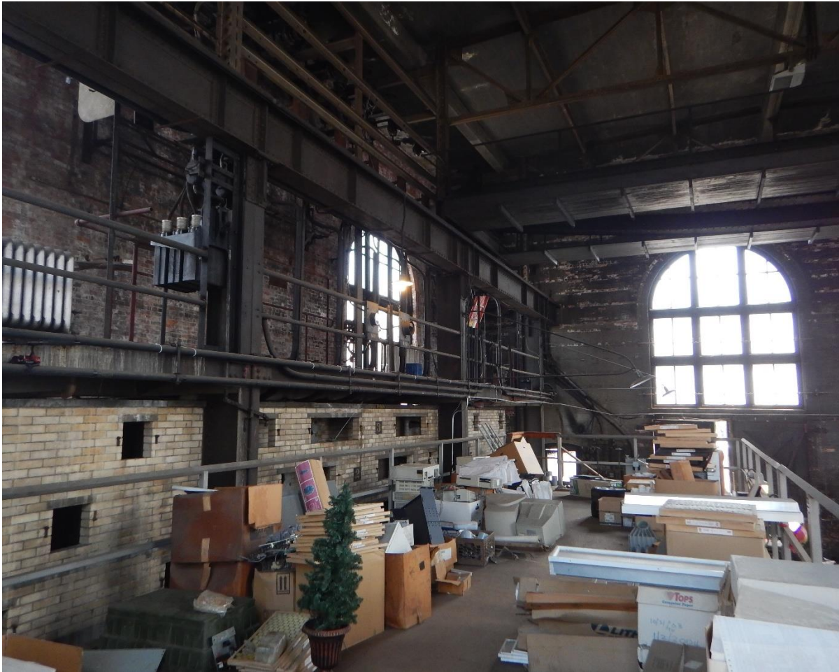
PHOTO 27. INTERIOR FACING SOUTHEAST
