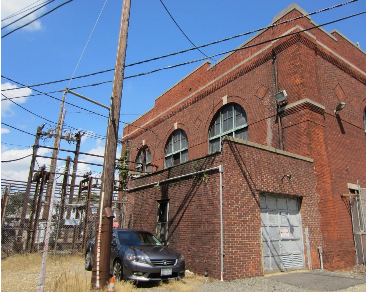
PHOTO 13. SOUTH AND WEST ELEVATIONS ADDITION
