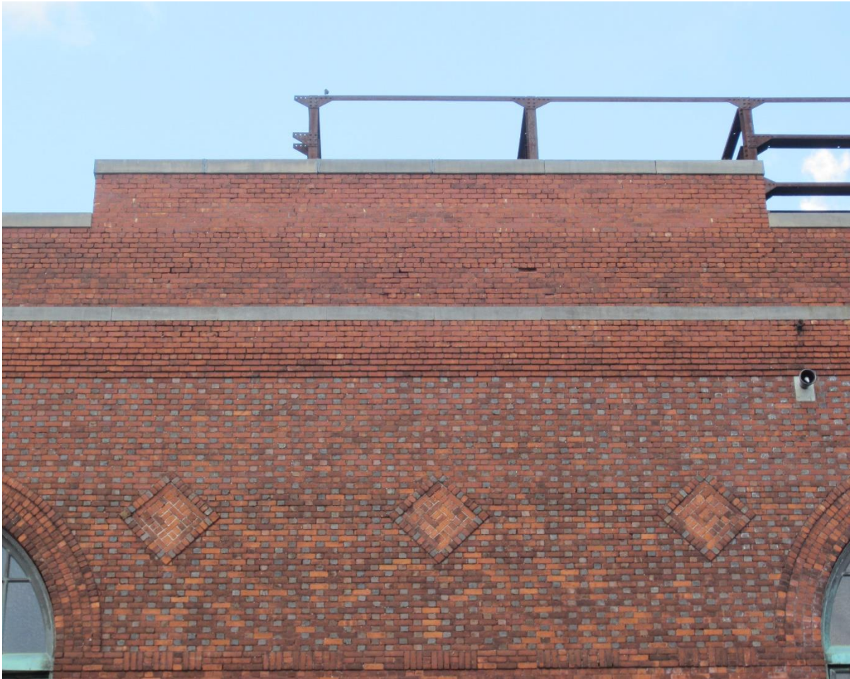
PHOTO 04. EAST ELEVATION BRICK DETAIL
