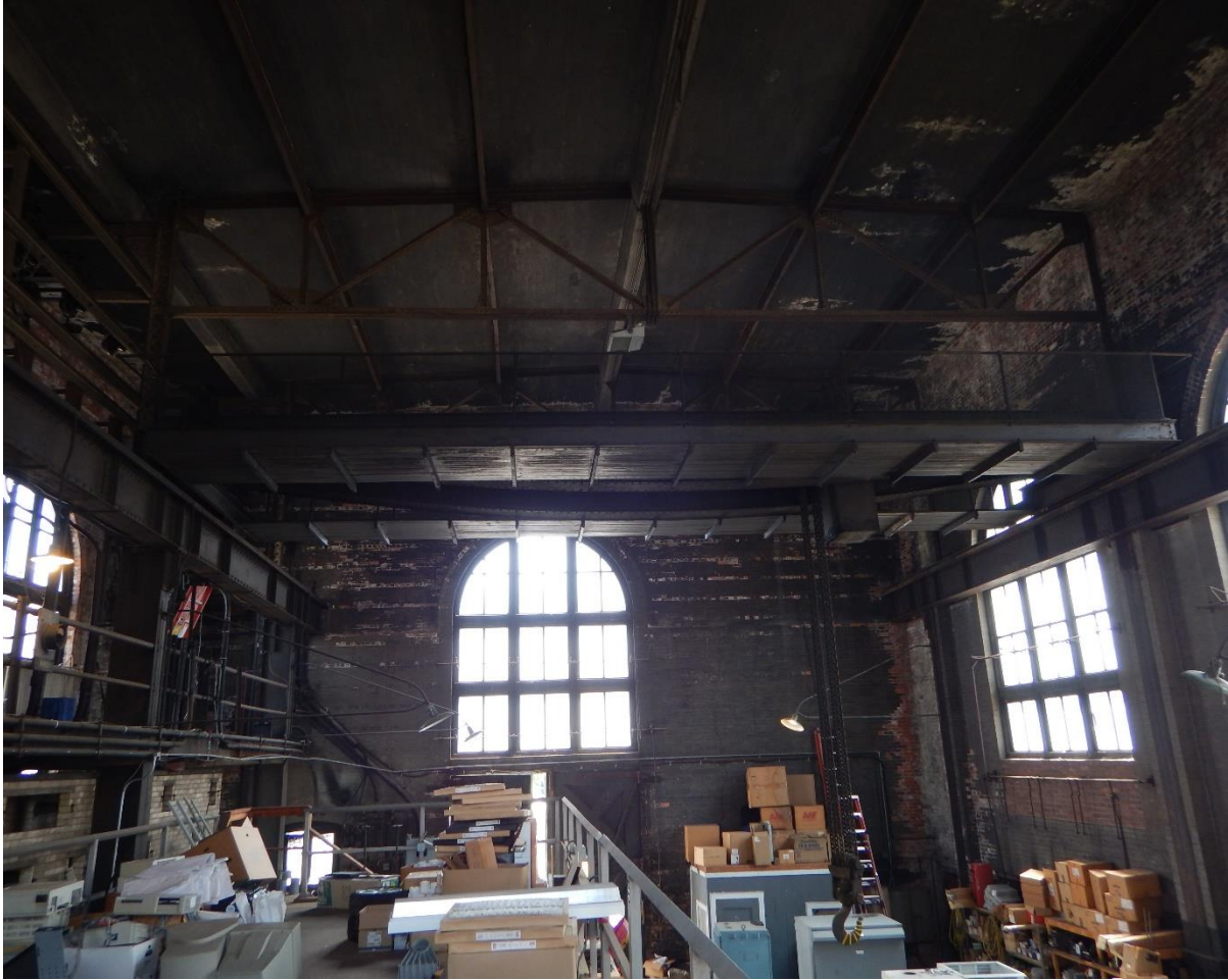
PHOTO 28. INTERIOR FACING SOUTH
