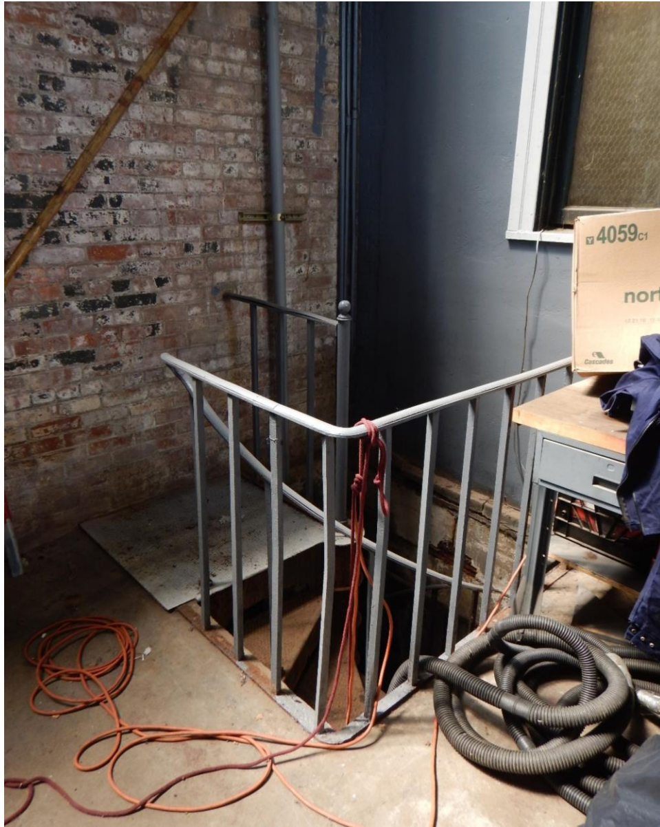
PHOTO 34. NORTHWEST SPIRAL STAIRCASE
