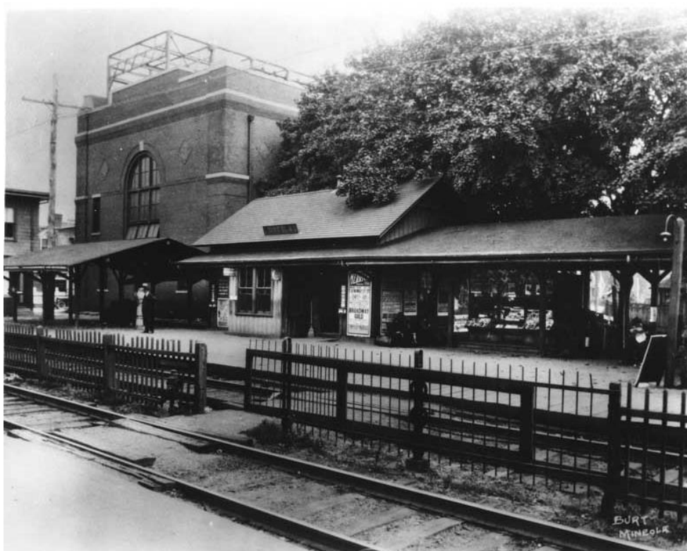
Fig.10. This post-1923 photograph shows how the 1883 station, signal tower (far left), and Electrical Substation are so close to each other that the east canopy of the station had to be moved to accommodate the substation. Source: Photographer Joe Burt, image accessed from the Queens Public Library.
