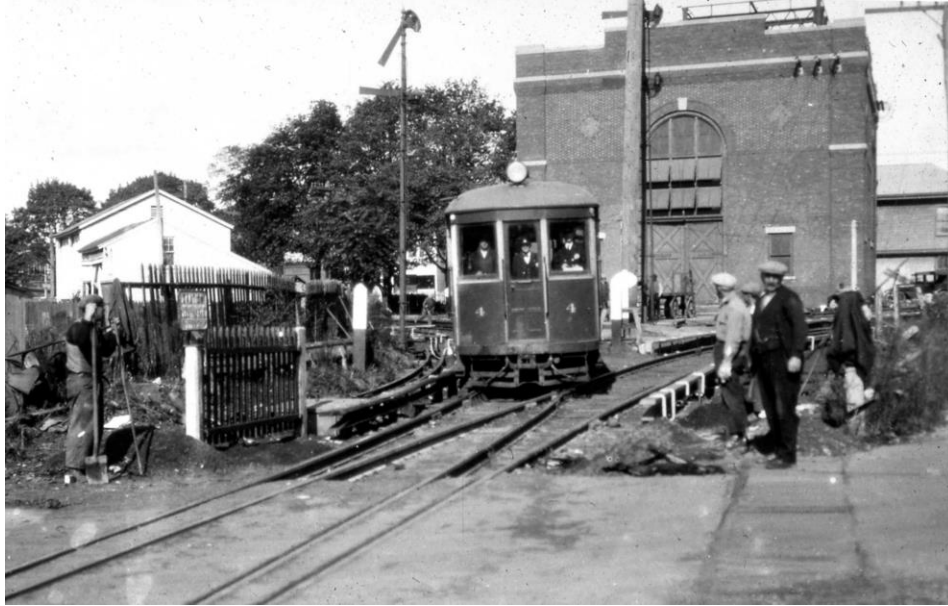
Fig. 11. Newly electrified rails in use around 1926, view looking north from the Hempstead Line tracks next to Main Street. The main doors and awning windows at the south facade of the Substation are clearly visible. Source: Huneke, Arthur John. "The L.I.R.R.'s Four Battery Cars." Last modified December 31, 2017. http://arrts-archives.com/battery.html . Image courtesy of Dave Keller.
