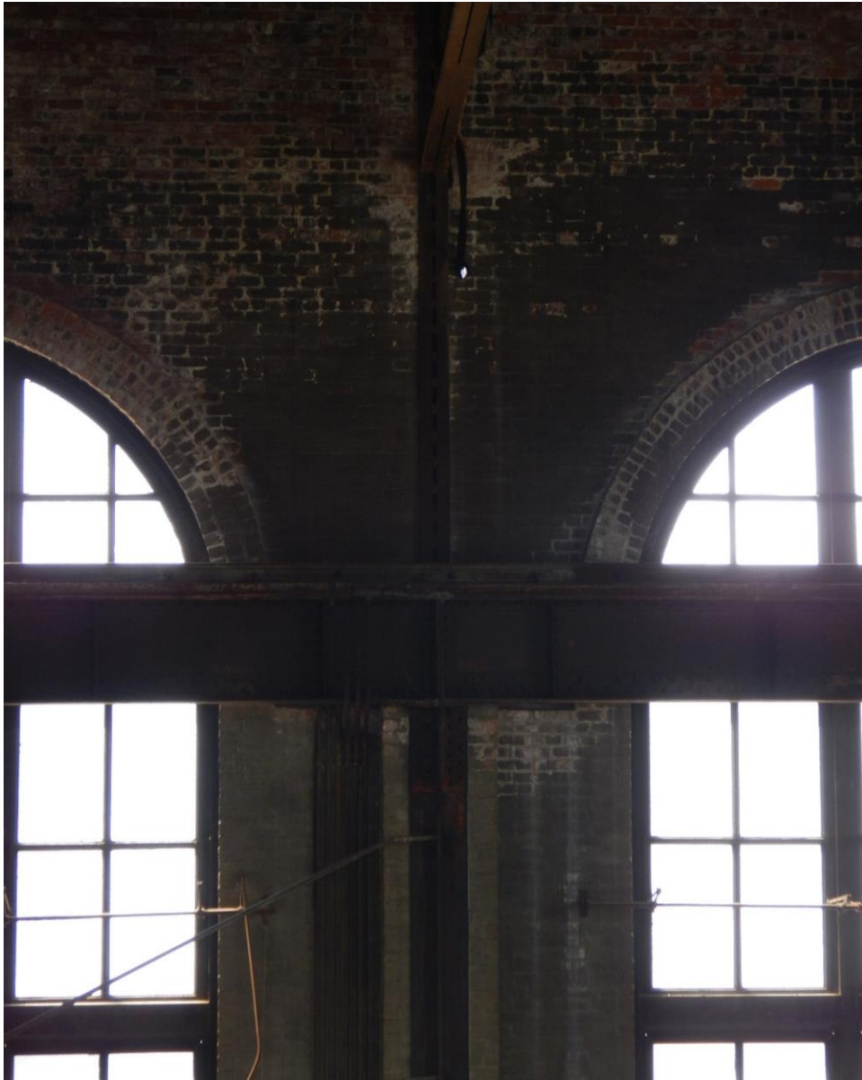
PHOTO 44. STEEL BEAM DETAIL
