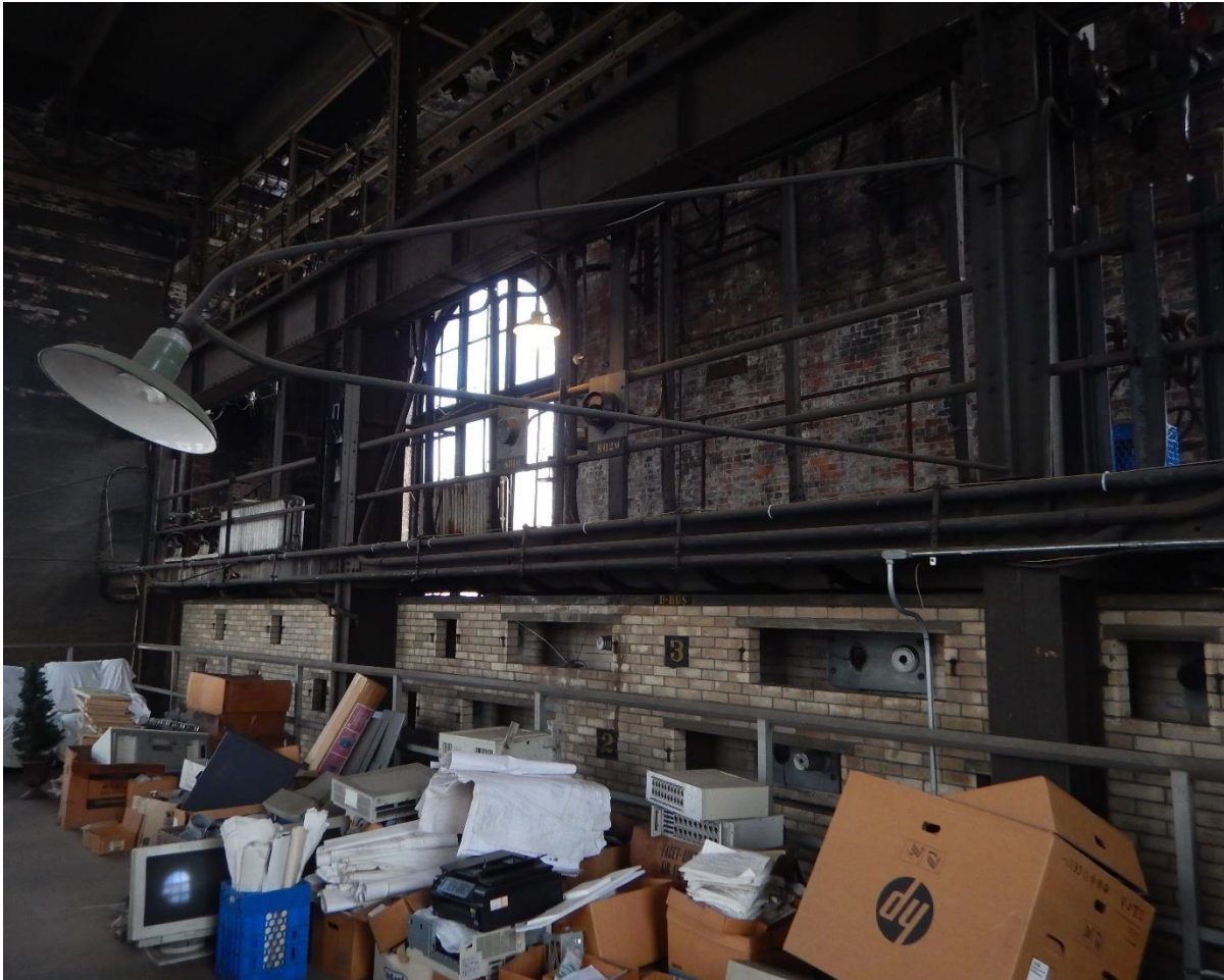
PHOTO 26. INTERIOR FACING NORTHEAST
