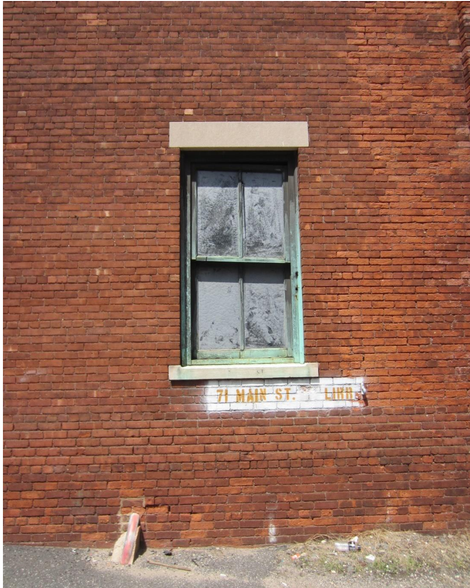
PHOTO 10. SOUTH ELEVATION WINDOW DETAIL
