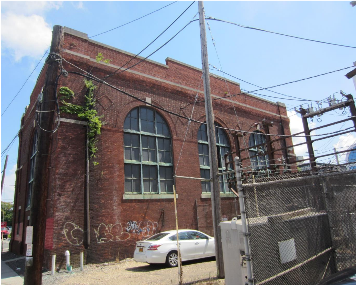
PHOTO 07. WEST ELEVATION OVERALL
