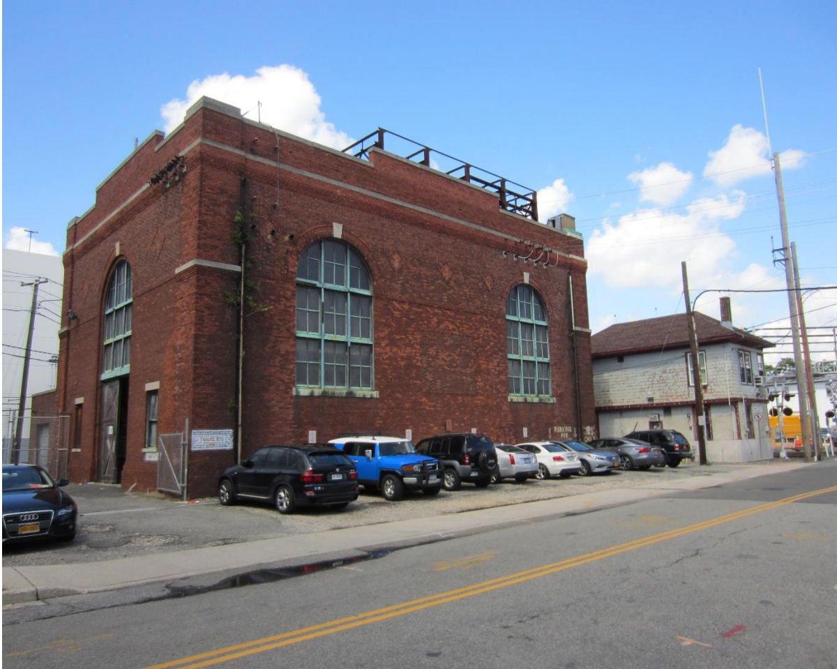
PHOTO 02. EAST AND SOUTH ELEVATIONS OVERALL
