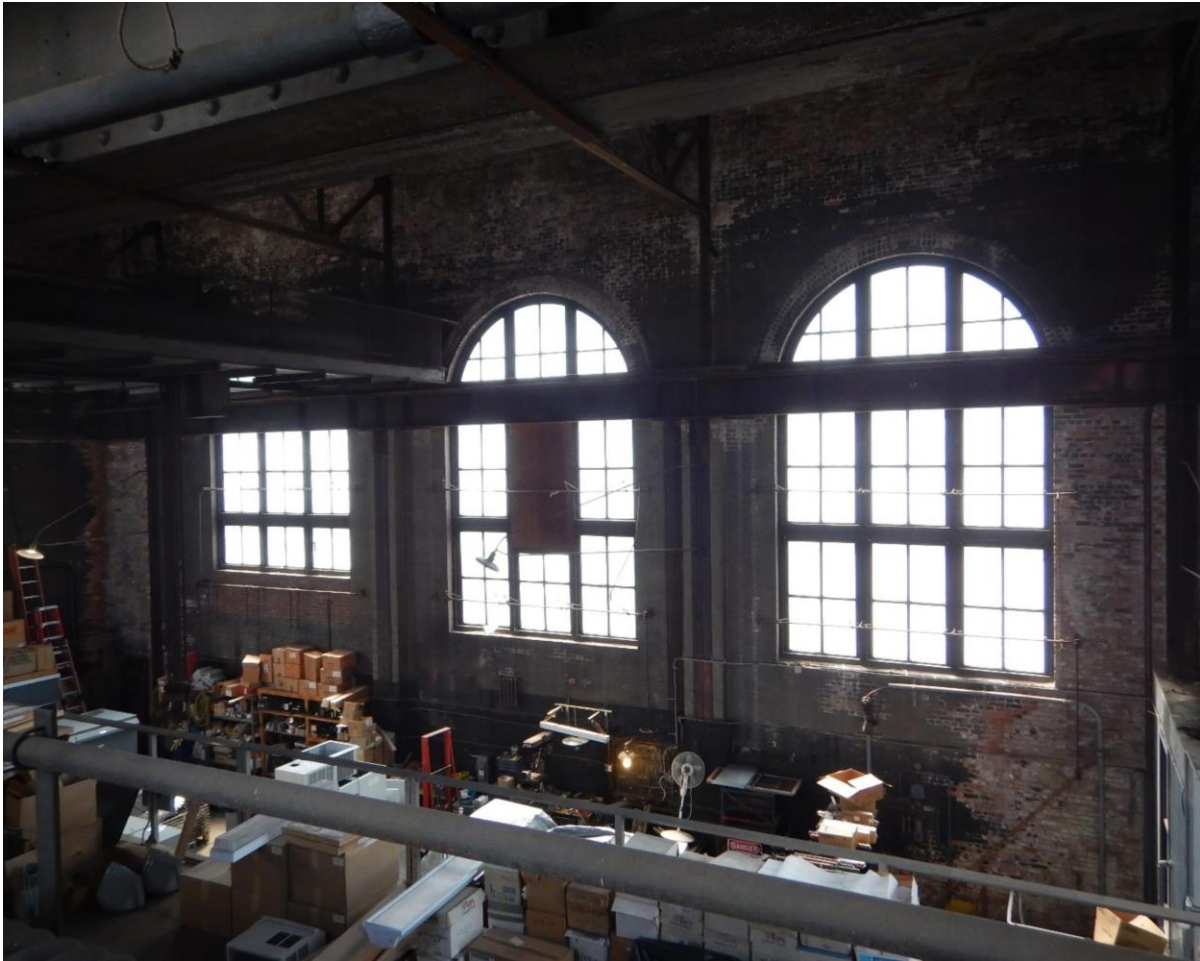
PHOTO 38. INTERIOR FACING WEST FROM MEZZANINE
