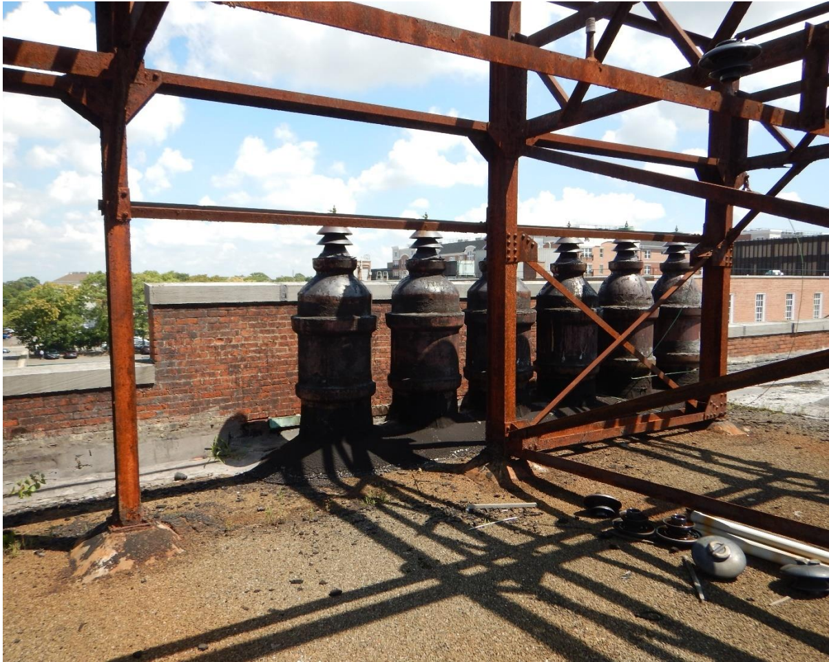
PHOTO 16. MAIN ROOF FACING EAST
