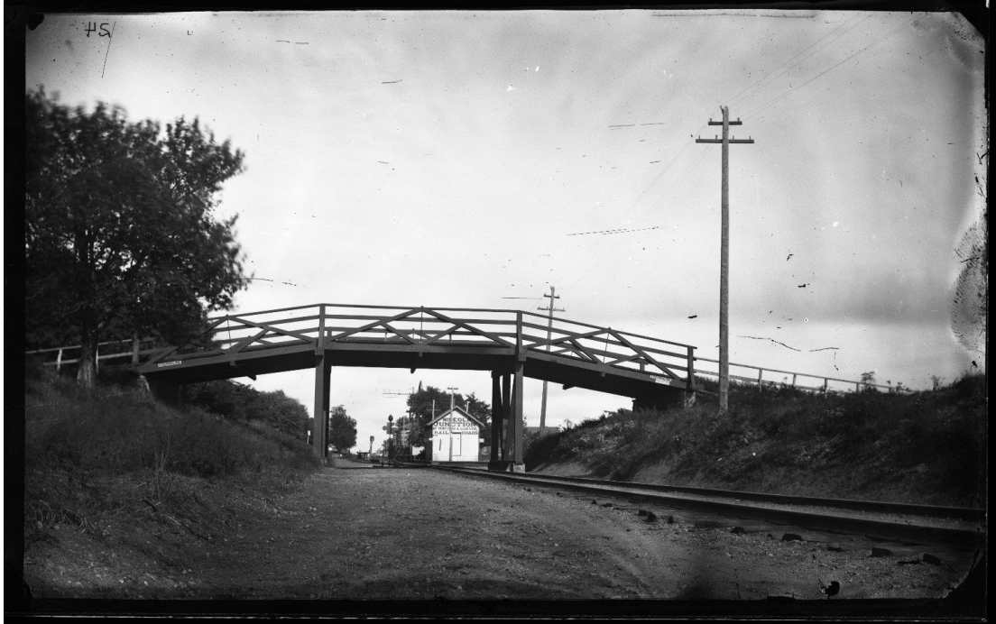
Fig. 4. An early grade-crossing elimination bridge carrying Mineola Boulevard. The Mineola station is visible in the distance beyond the bridge. Source: Brainerd, George Bradford. Bridge, Mineola, Long Island . 1872-1887. Collodion silver glass wet plate negative. Image courtesy of the Brooklyn Museum, https://www.brooklynmuseum.org/opencollection/objects/191059 .
