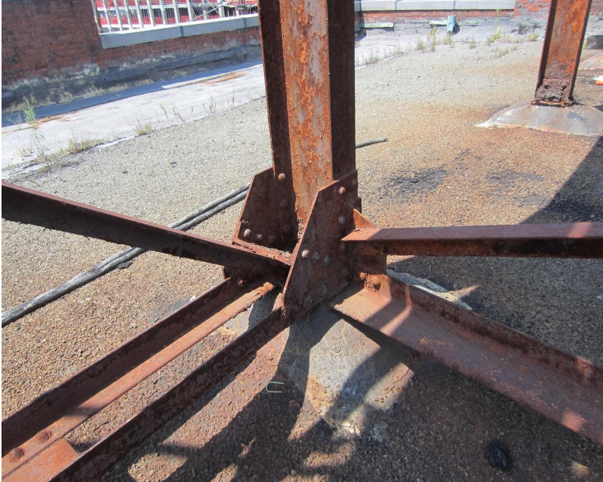
PHOTO 22. MAIN ROOF STEEL STRUCTURE
