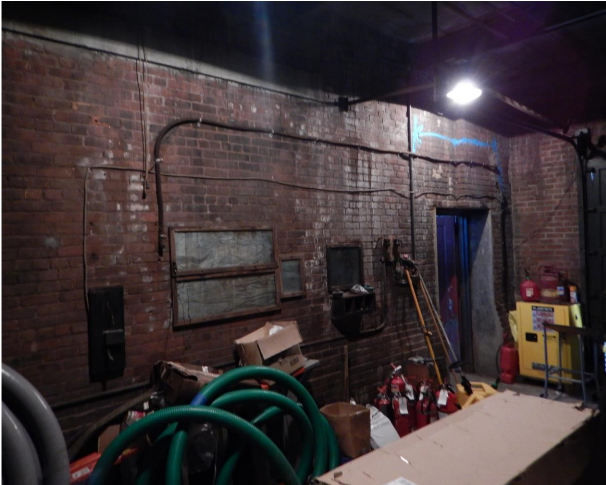
PHOTO 53. INTERIOR ADDITION FACING SOUTHEAST
