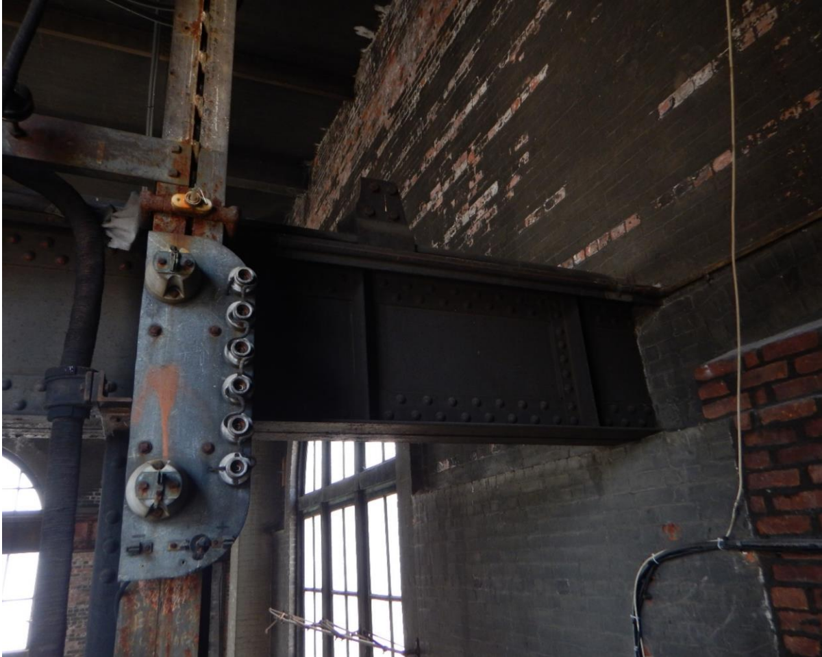
PHOTO 46. STEEL BEAM DETAIL
