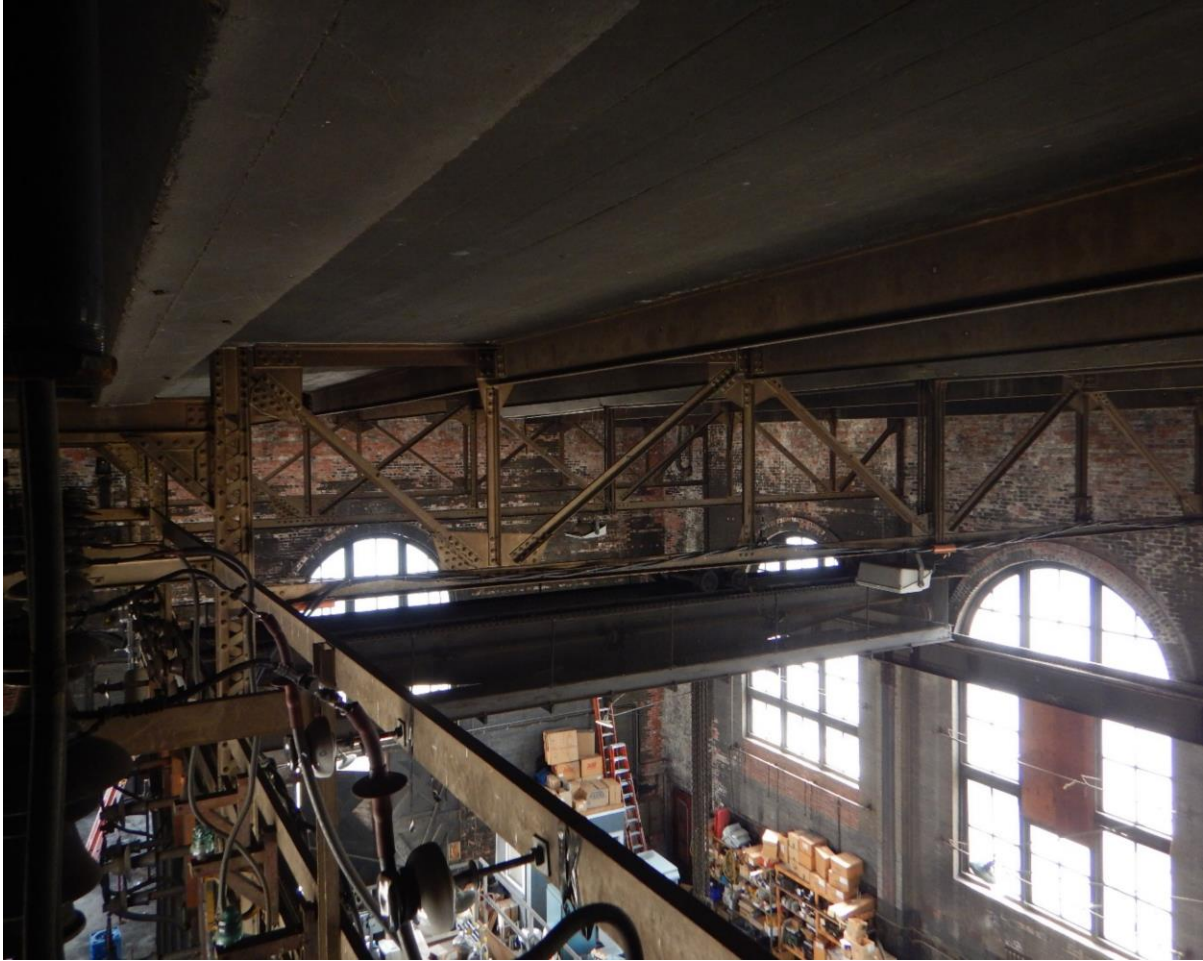
PHOTO 50. STEEL TRUSS DETAIL
