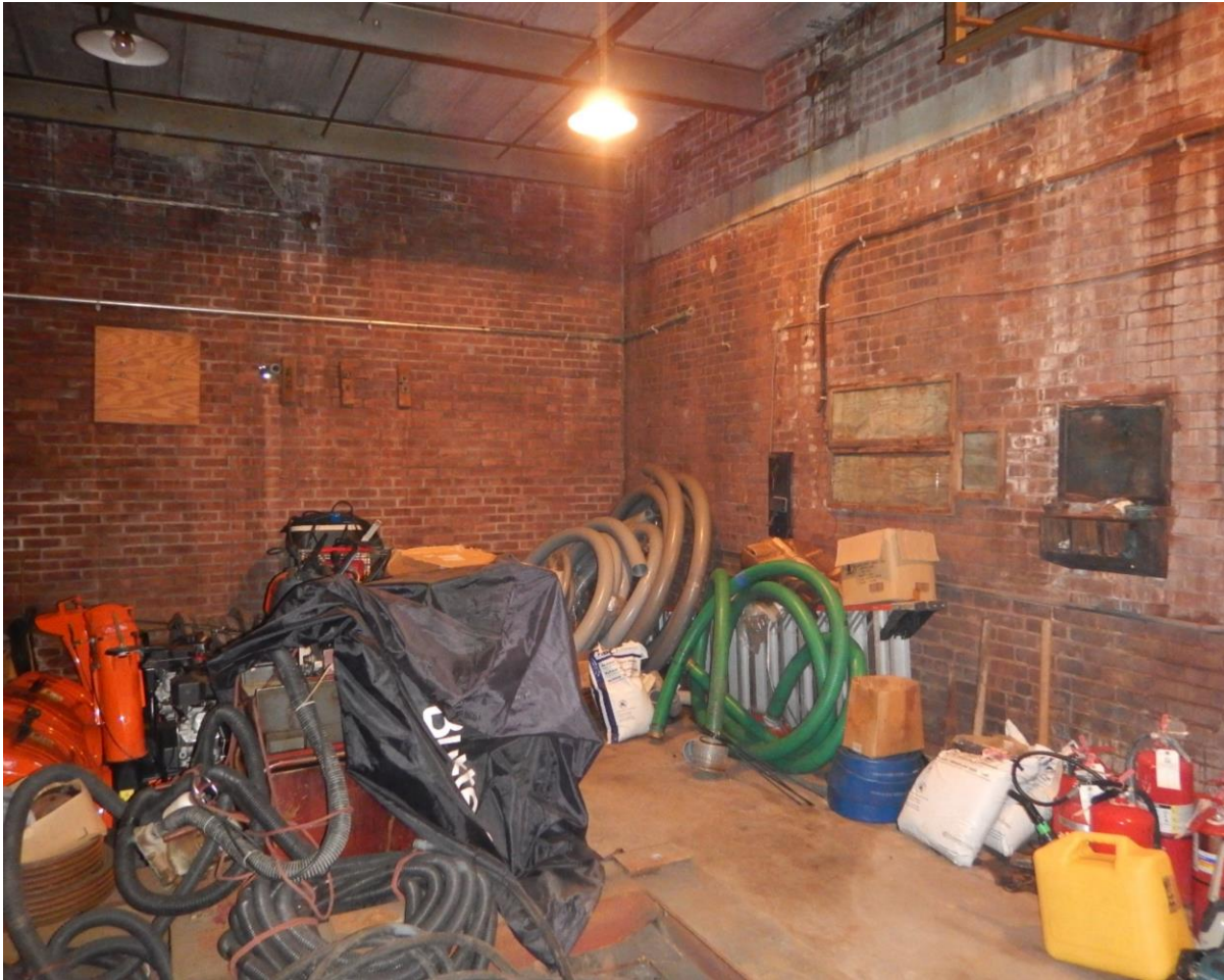
PHOTO 52. INTERIOR ADDITION FACING NORTHEAST
