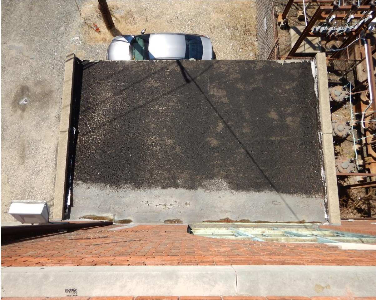
PHOTO 23. ROOF OF ADDITION
