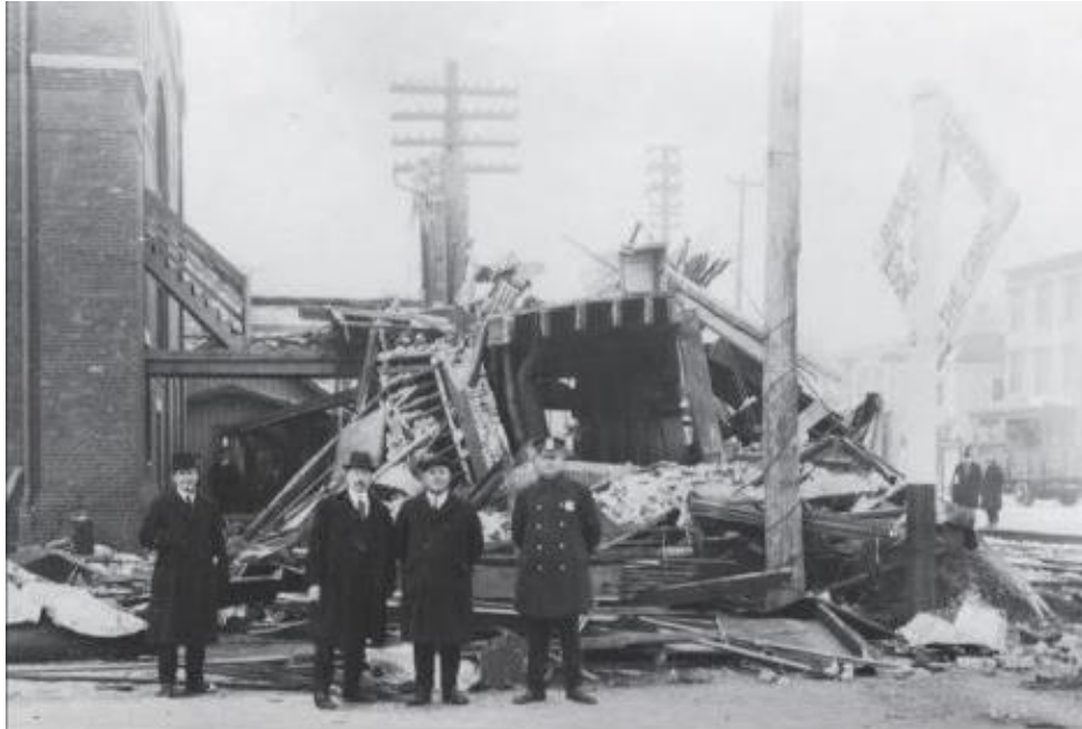
Fig. 9. The destroyed brick signal tower would be replaced by the Nassau Tower in 1923. The platform and stair that connected the tower and the Substation is clearly visible at left. These were likely demolished around the time of the new tower's construction. Source: Long Island Rail Road: Oyster Bay Branch , 28.
