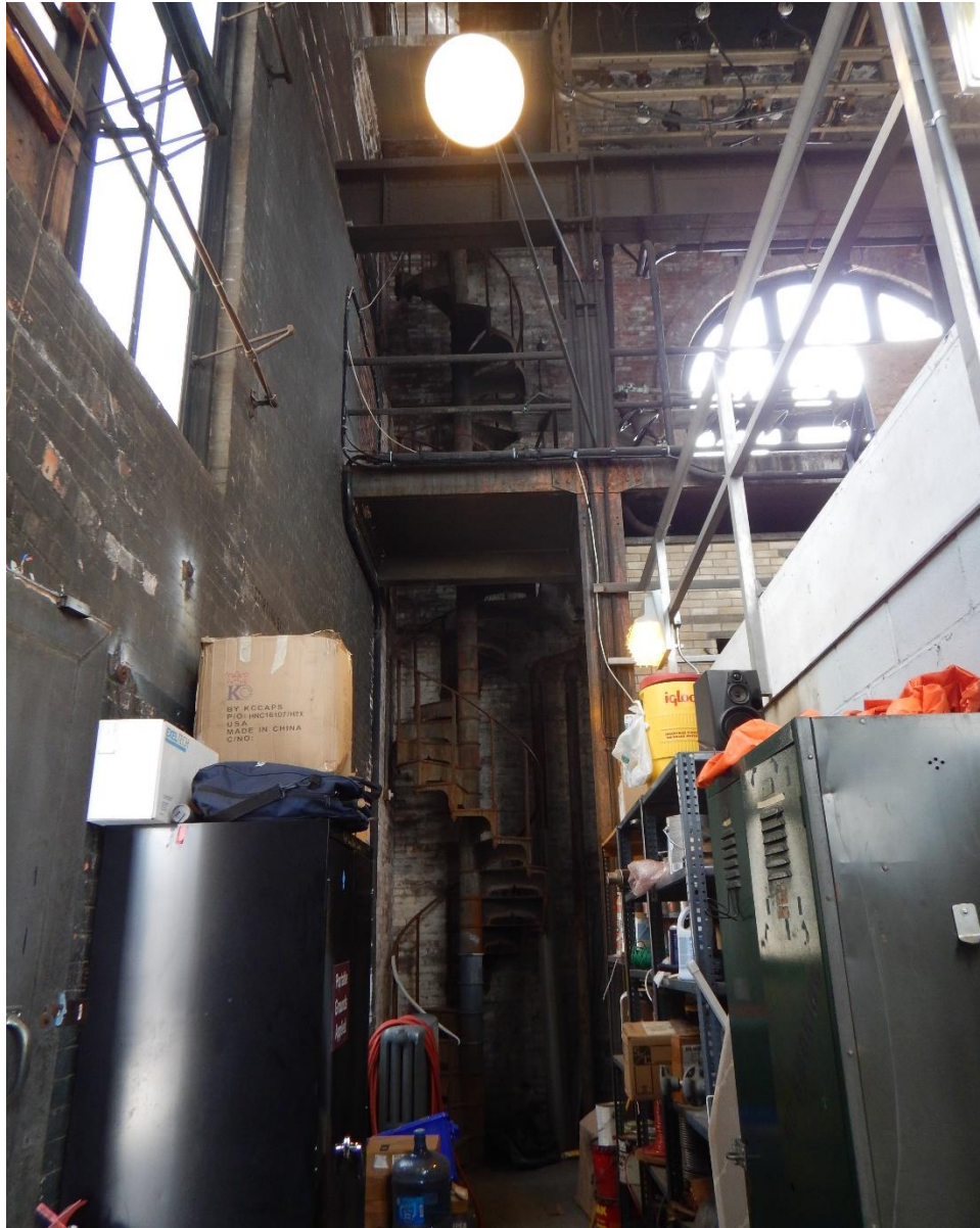
PHOTO 32. NORTHEAST SPIRAL STAIRCASE
