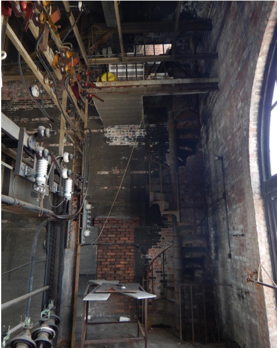
PHOTO 45. NORTHEAST SPIRAL STAIRCASE
