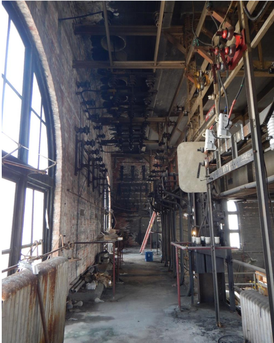
PHOTO 37. MEZZANINE FACING SOUTH
