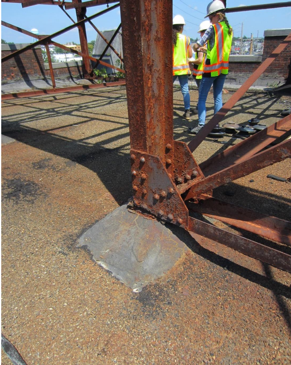
PHOTO 20. MAIN ROOF STEEL STRUCTURE
