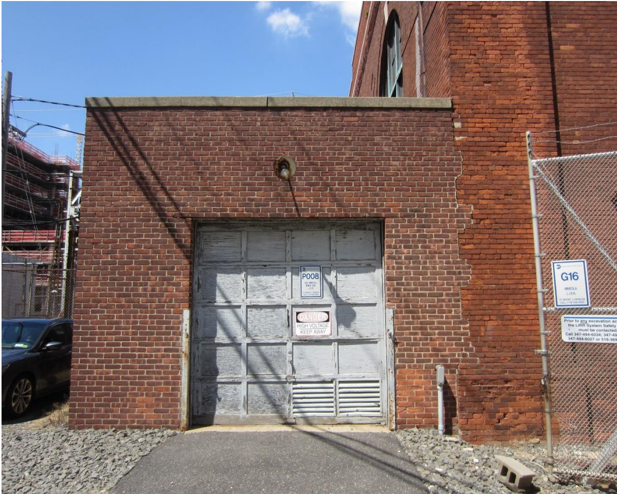
PHOTO 12. SOUTH ELEVATION ADDITION
