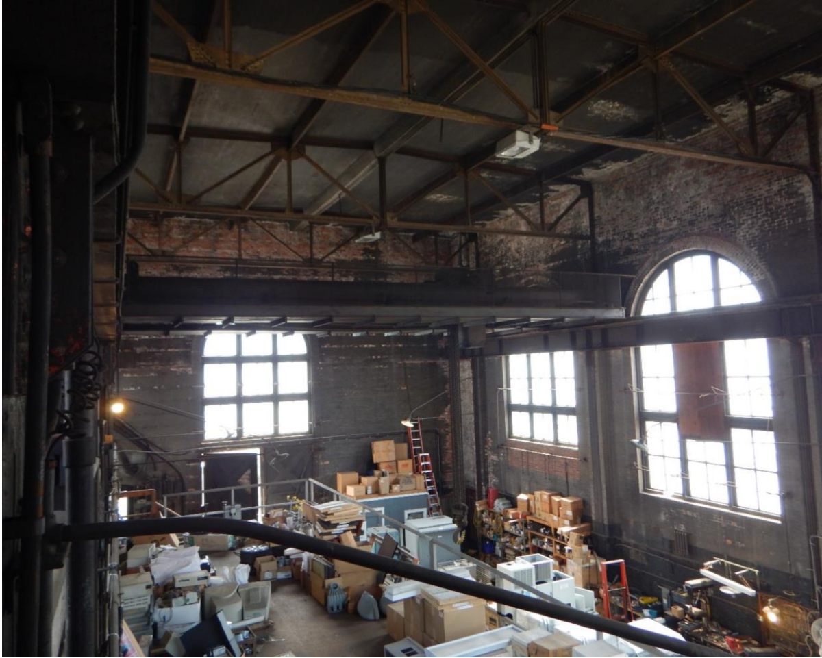
PHOTO 39. INTERIOR FACING SOUTHWEST FROM MEZZANINE
