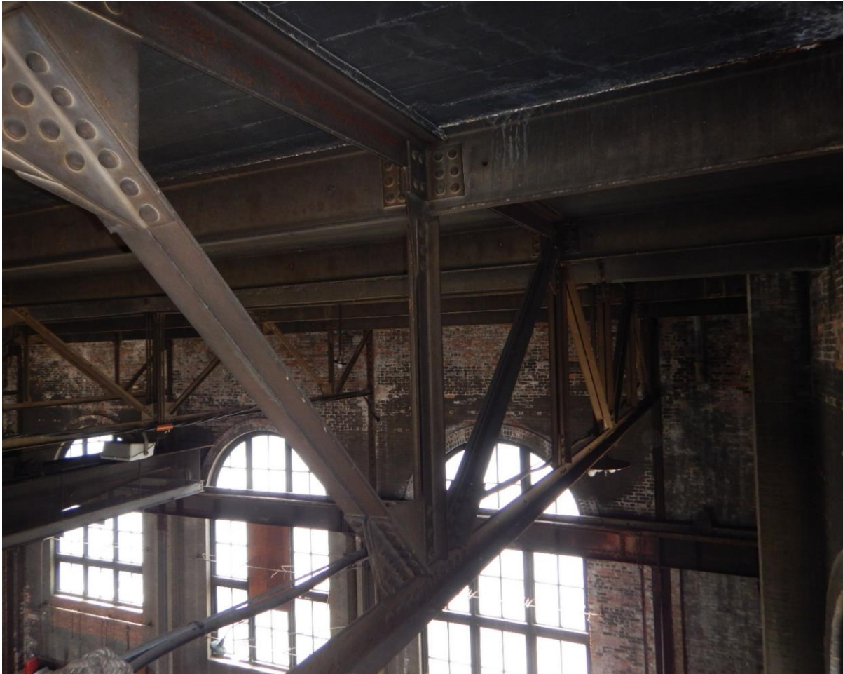
PHOTO 48. STEEL TRUSS DETAIL
