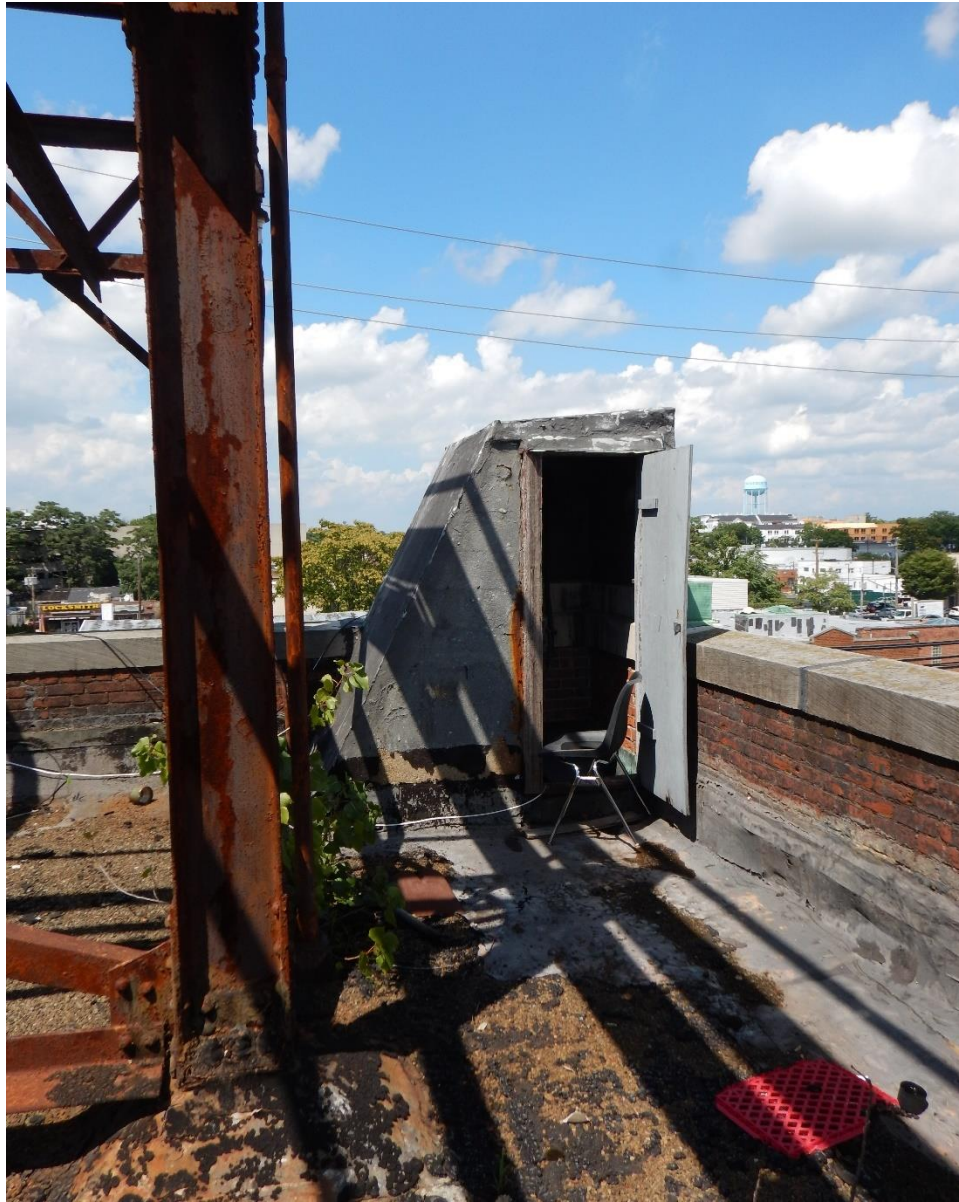
PHOTO 17. MAIN ROOF STAIR BULKHEAD
