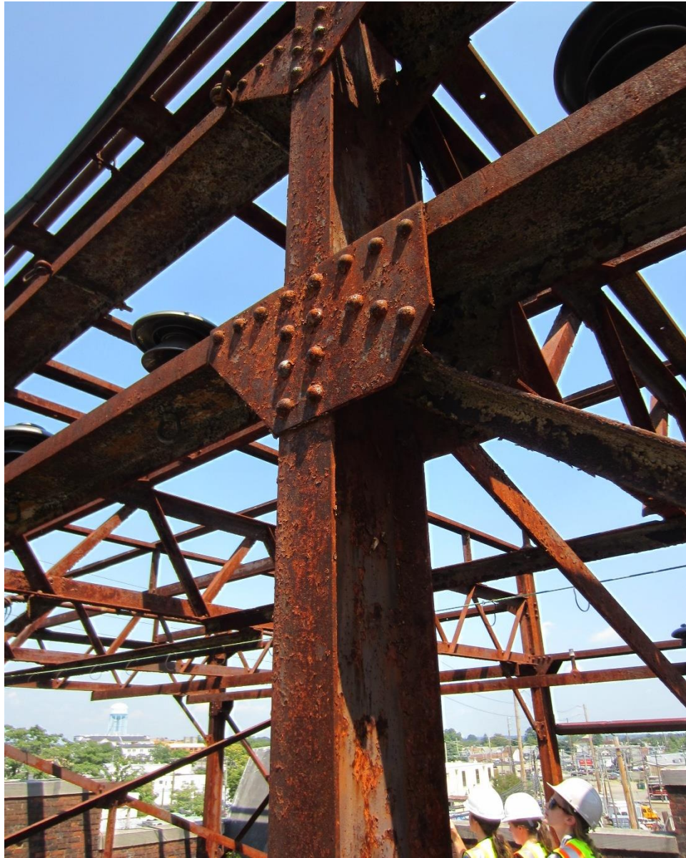
PHOTO 21. MAIN ROOF STEEL STRUCTURE
