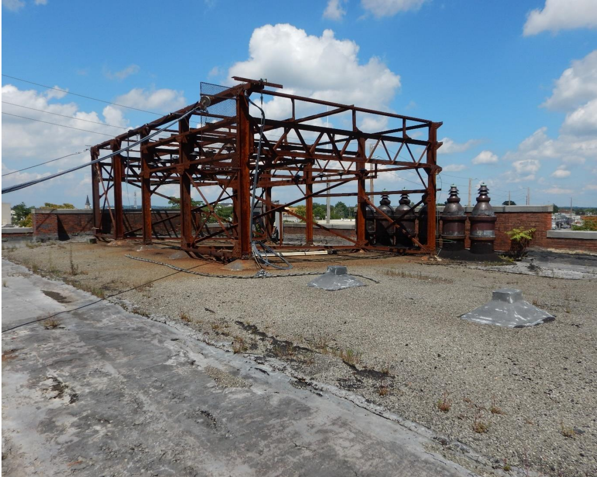
PHOTO 18. MAIN ROOF FACING NORTHEAST
