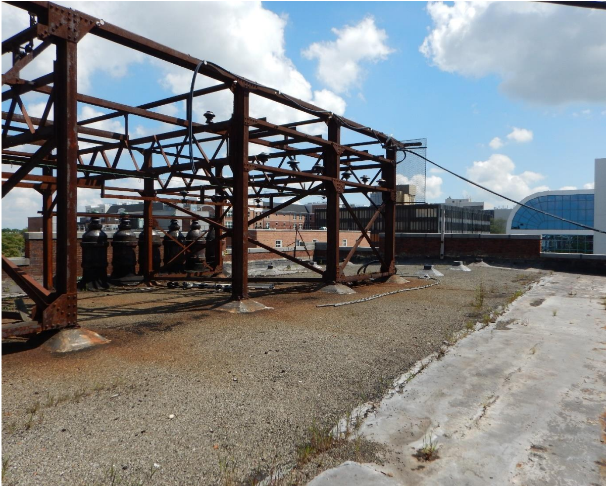
PHOTO 19. MAIN ROOF FACING SOUTHEAST
