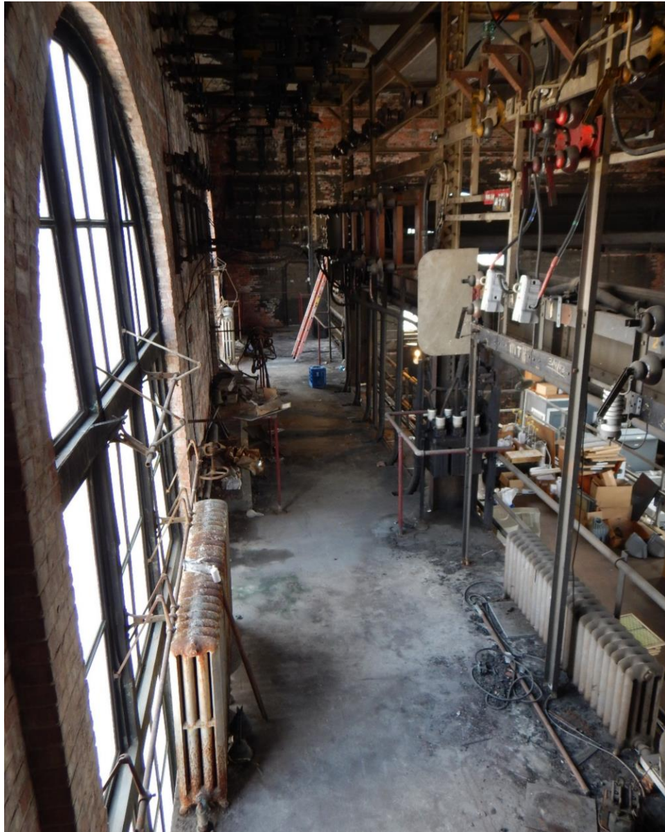
PHOTO 47. MEZZANINE FACING SOUTH
