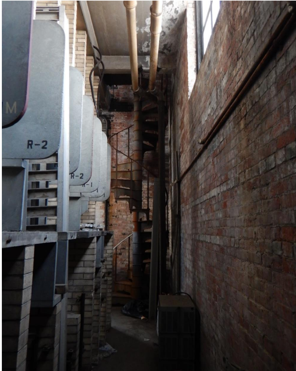
PHOTO 36. NORTHEAST SPIRAL STAIRCASE
