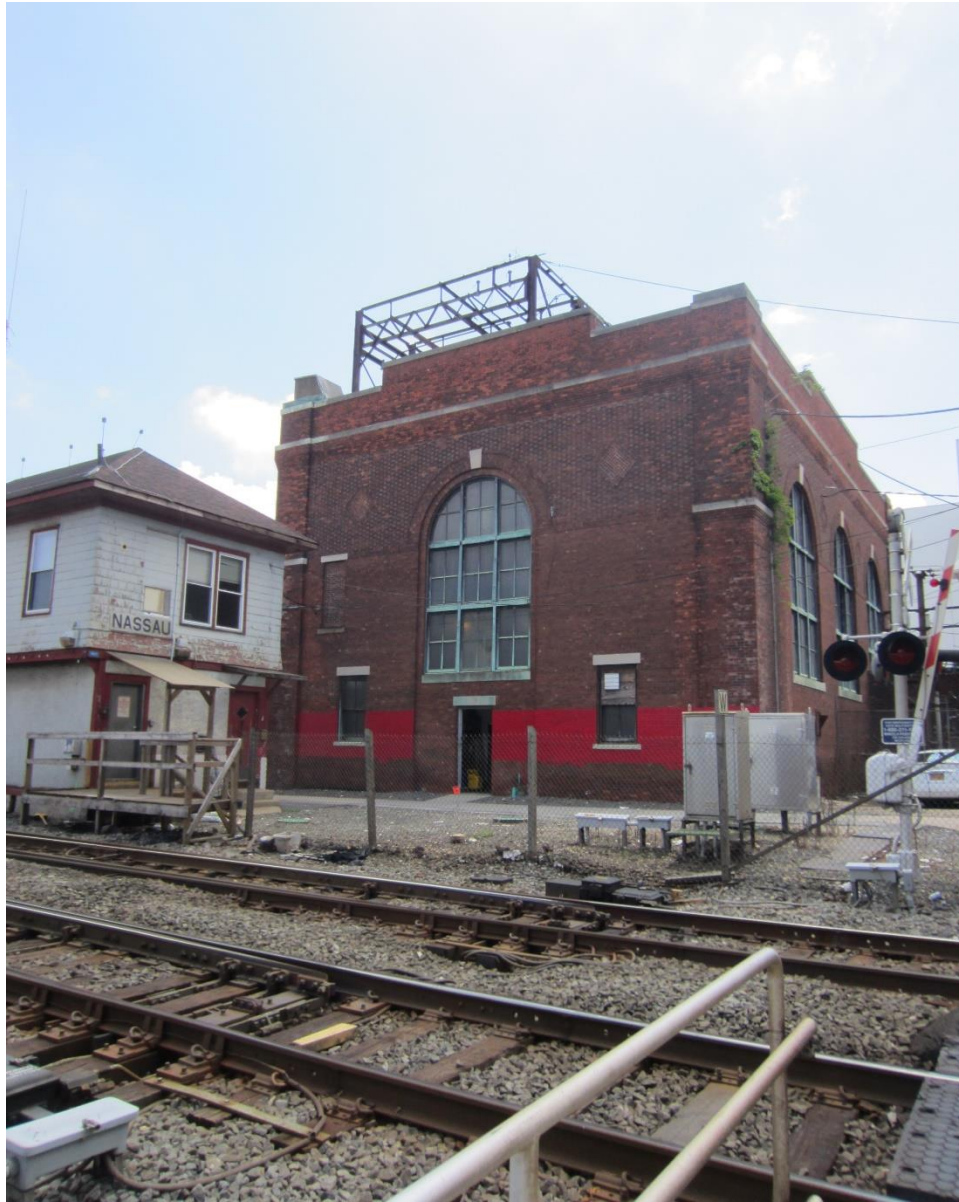
PHOTO 06. NORTH ELEVATION OVERALL
