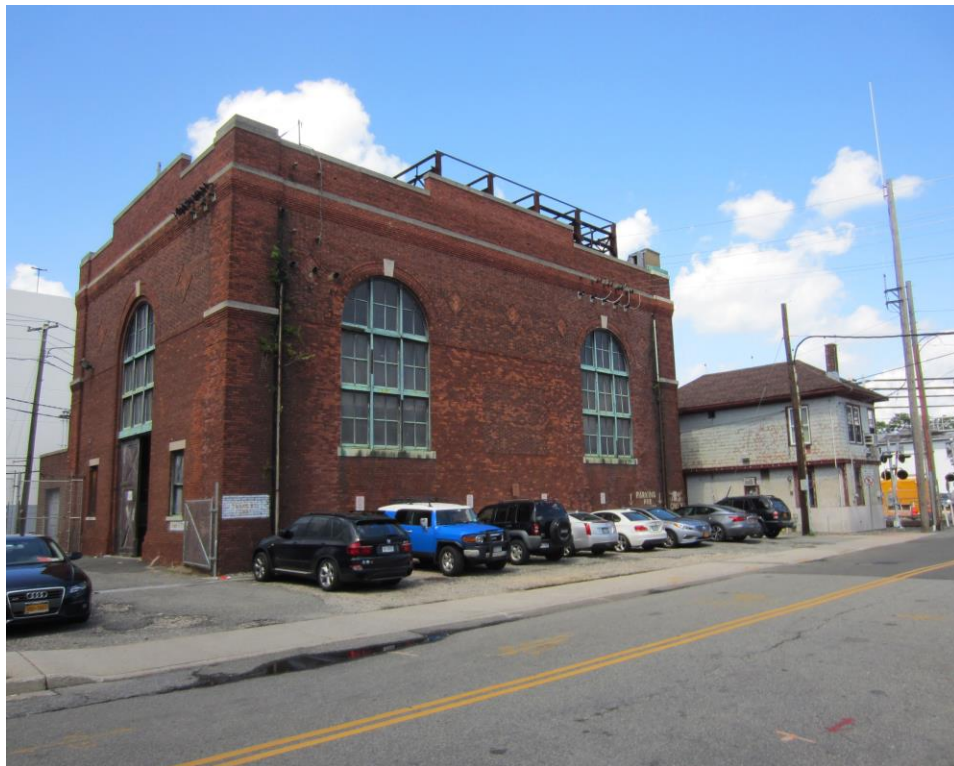
The former Mineola LIRR Electrical Substation, August 14, 2018.
