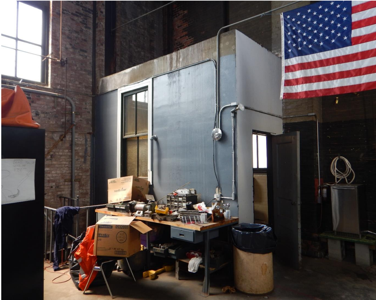
PHOTO 31. NORTHWEST CORNER BATHROOM ADDITION
