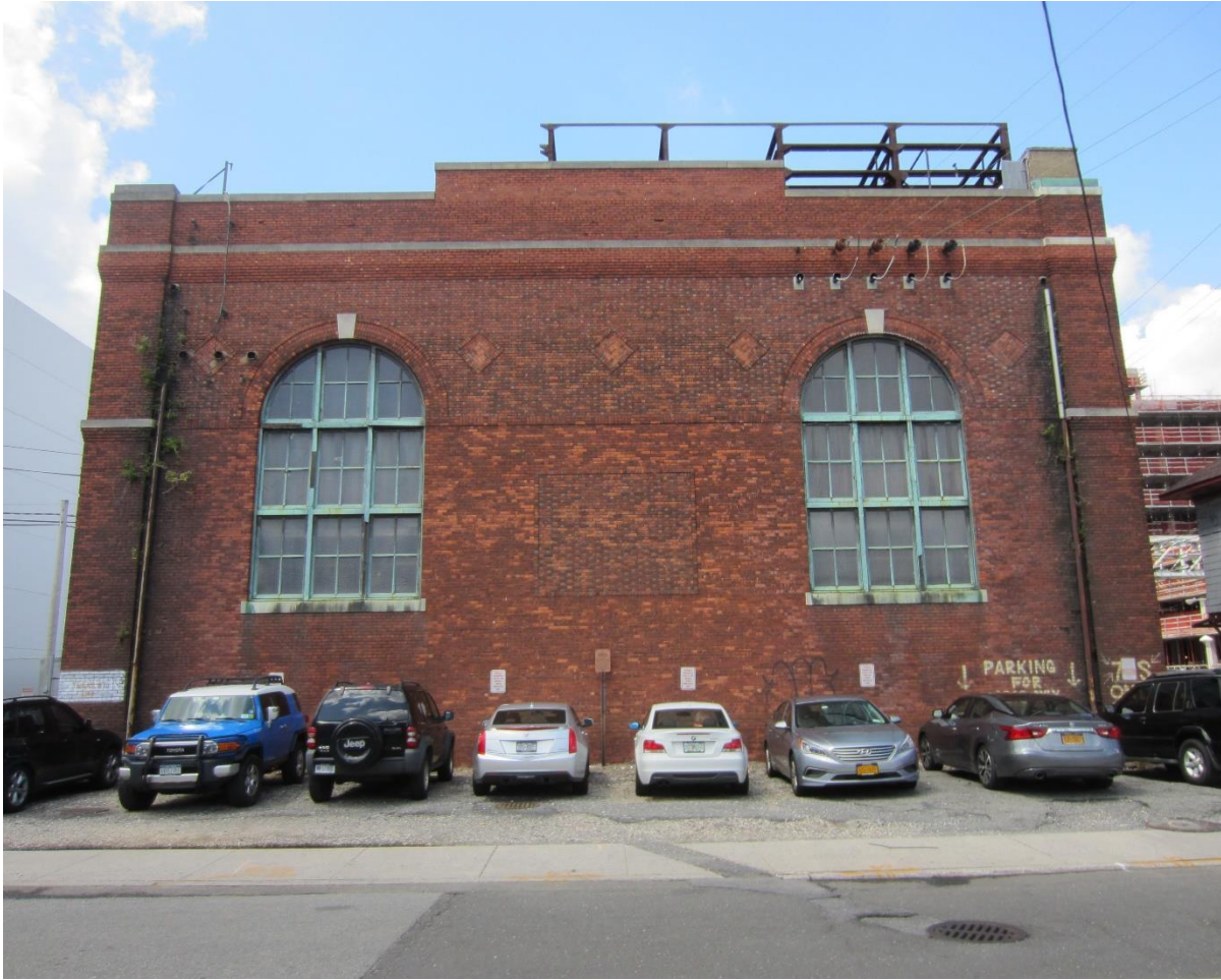
PHOTO 01. EAST ELEVATION OVERALL
