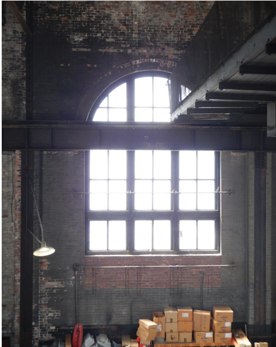
PHOTO 41. WEST WALL WINDOW DETAIL
