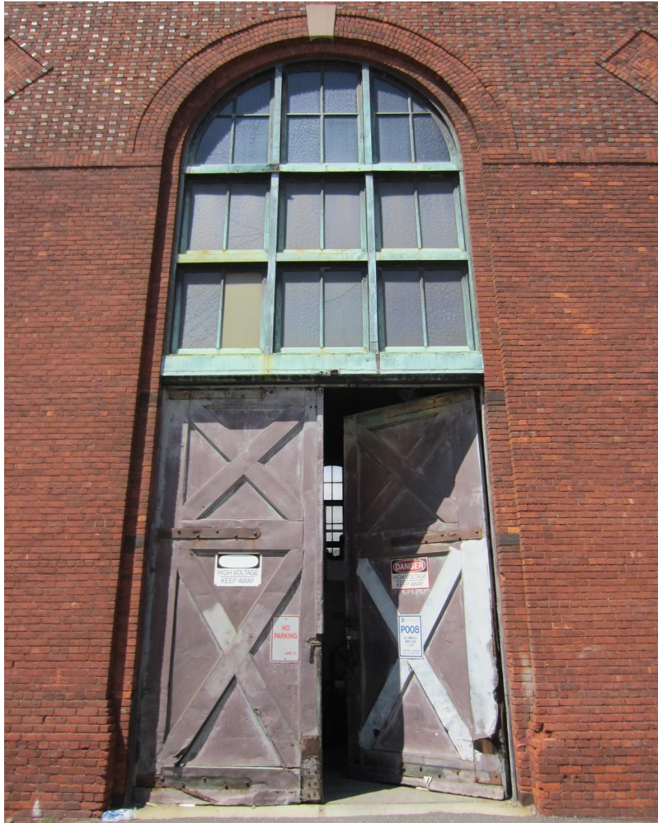
PHOTO 09. SOUTH ELEVATION ENTRY DOOR DETAIL
