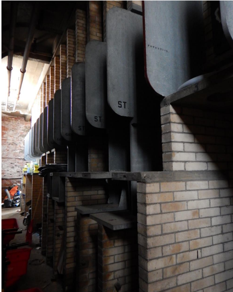
PHOTO 35. AREA UNDER MEZZANINE
