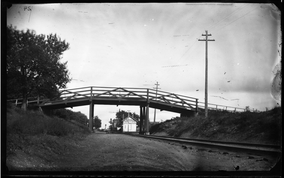
Fig. 4. An early grade-crossing elimination bridge carrying Mineola Boulevard. The Mineola station is visible in the distance beyond the bridge. Source: Brainerd, George Bradford. Bridge, Mineola, Long Island . 1872-1887. Collodion silver glass wet plate negative. Image courtesy of the Brooklyn Museum, https://www.brooklynmuseum.org/opencollection/objects/191059 .
