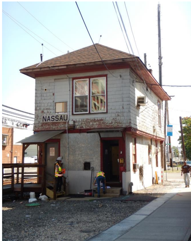
The Nassau Tower, August 14, 2018.
