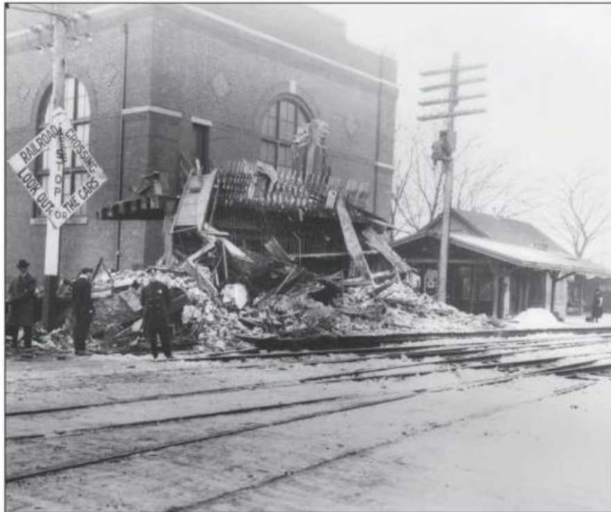
Fig. 8. The brick signal tower was destroyed on December 31, 1922. The north and east facades of the Substation are unharmed, viewed looking south on Main Street. Source: Long Island Rail Road: Oyster Bay Branch, 29 .
