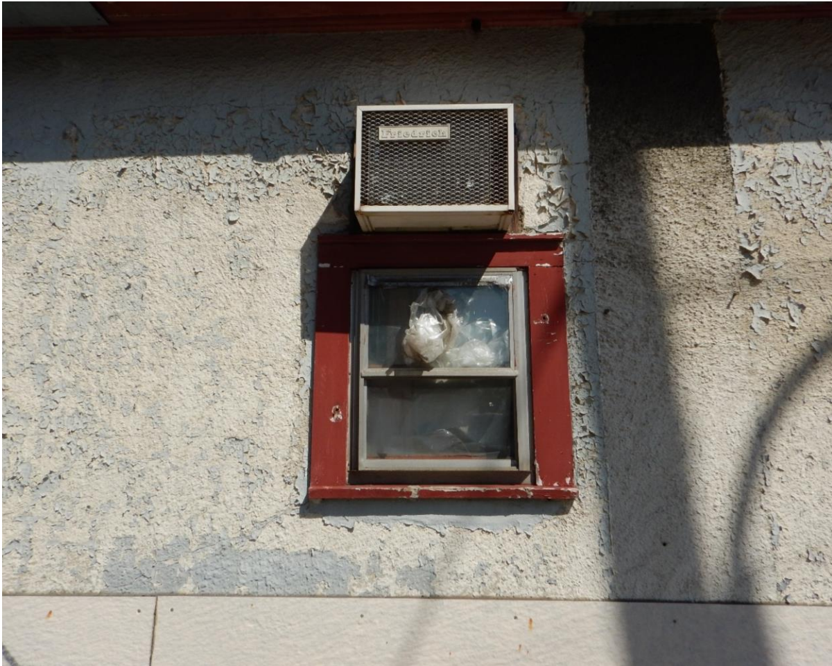
PHOTO 60. SOUTH ELEVATION WINDOW DETAIL
