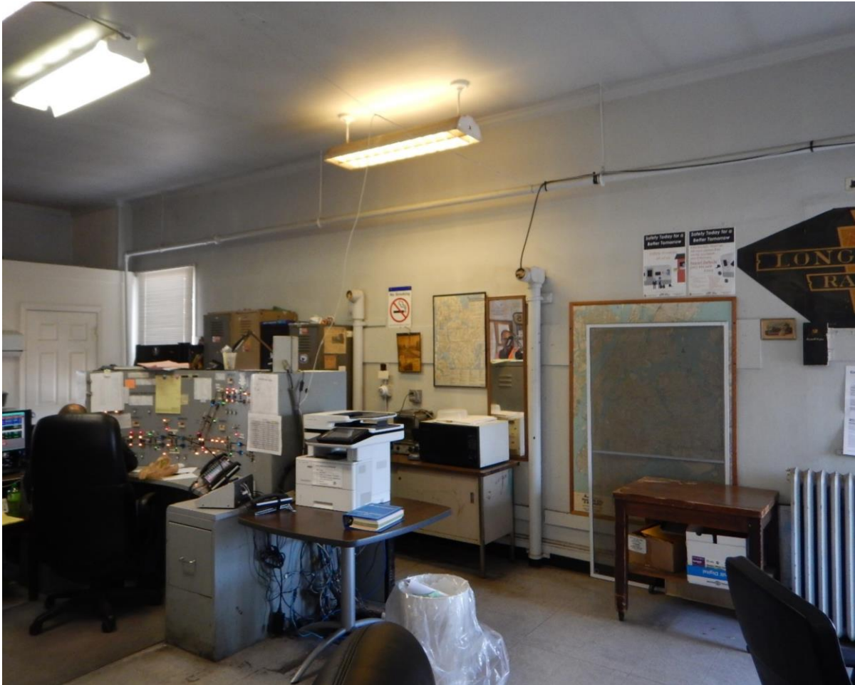
PHOTO 82. SECOND FLOOR FACING NORTH
