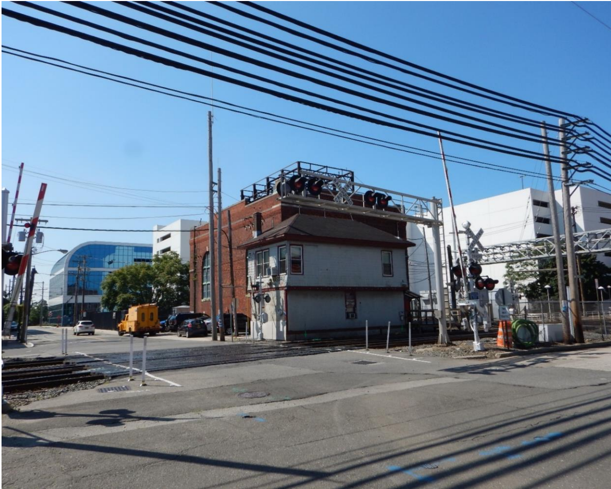
PHOTO 58. NORTH AND EAST ELEVATIONS OVERALL
