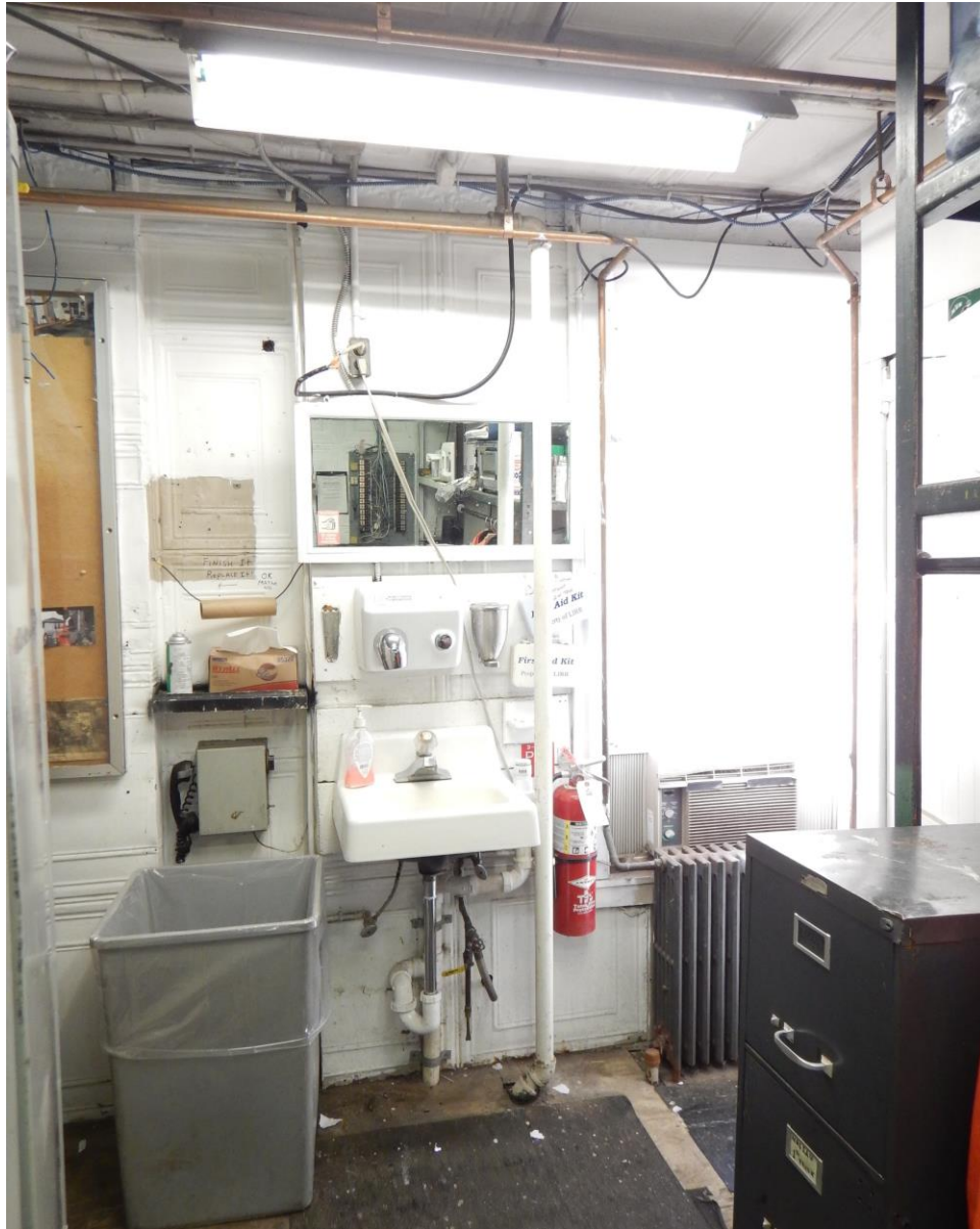
PHOTO 67. FIRST FLOOR FACING SOUTH
