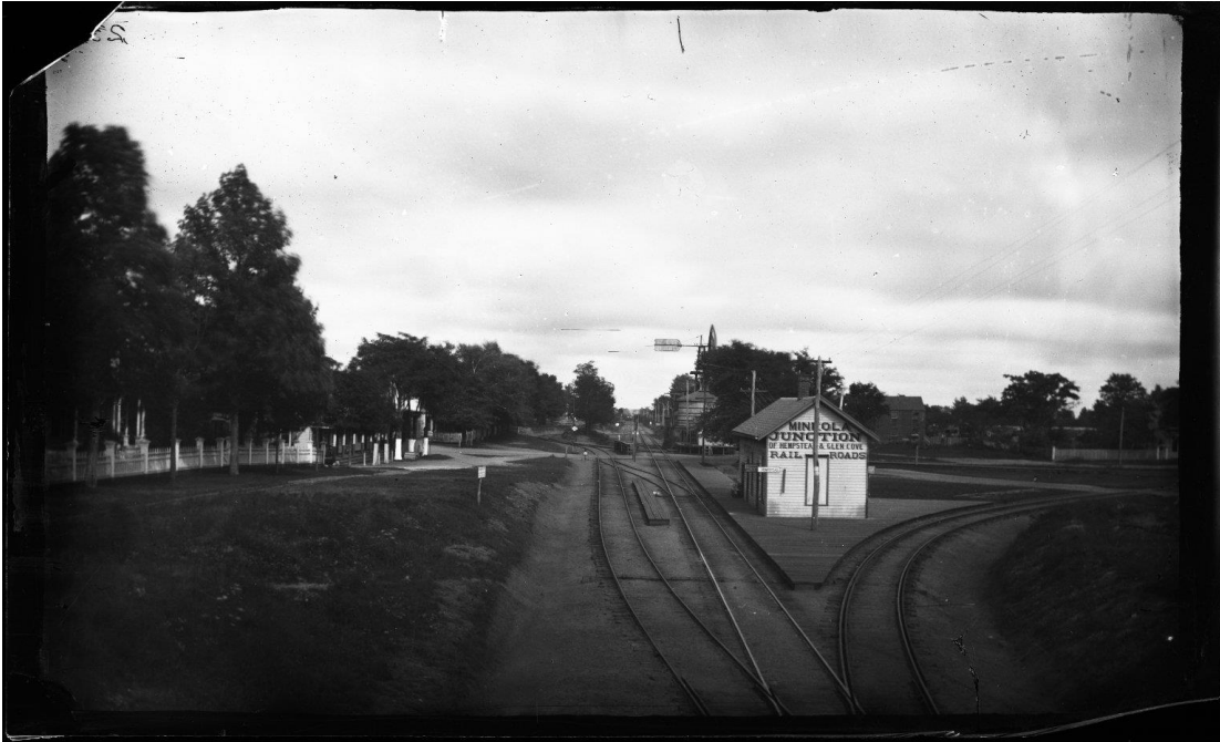
Fig. 3. View of an early Mineola Station, c.1872-1887, looking east along the Main Line tracks. The Hempstead Branch line (right) turns southward. Source: Brainerd, George Bradford. Mineola Station, Long Island . 1872-1887. Collodion silver glass wet plate negative. Image courtesy of the Brooklyn Museum, https://www.brooklynmuseum.org/opencollection/objects/191058 .
