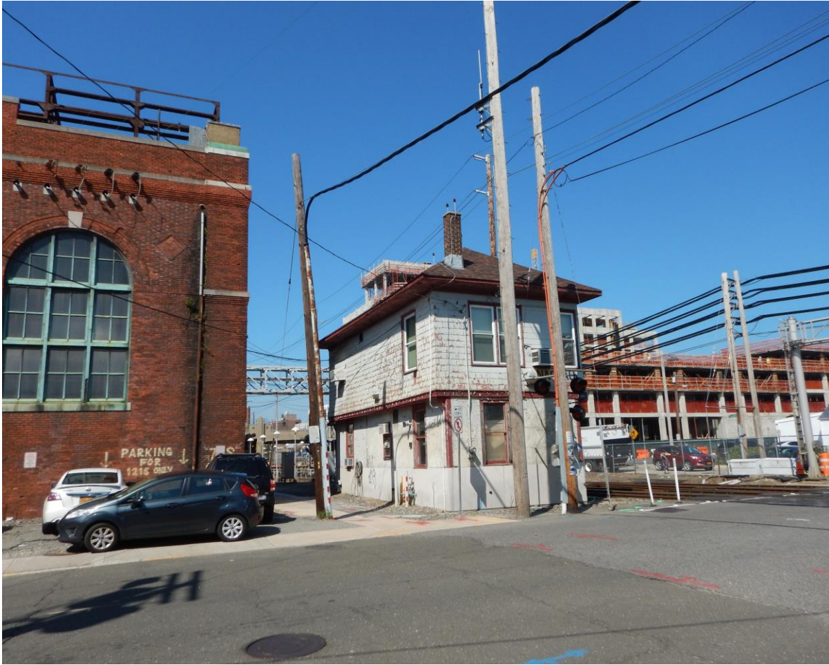
PHOTO 54. SOUTH AND EAST ELEVATIONS OVERALL
