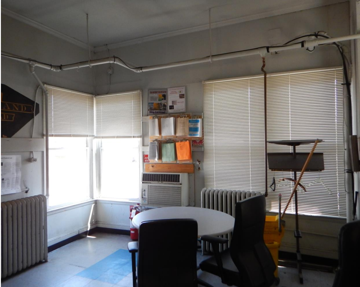
PHOTO 81. SECOND FLOOR FACING NORTHEAST
