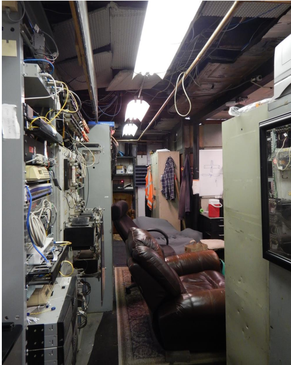
PHOTO 68. FIRST FLOOR FACING EAST
