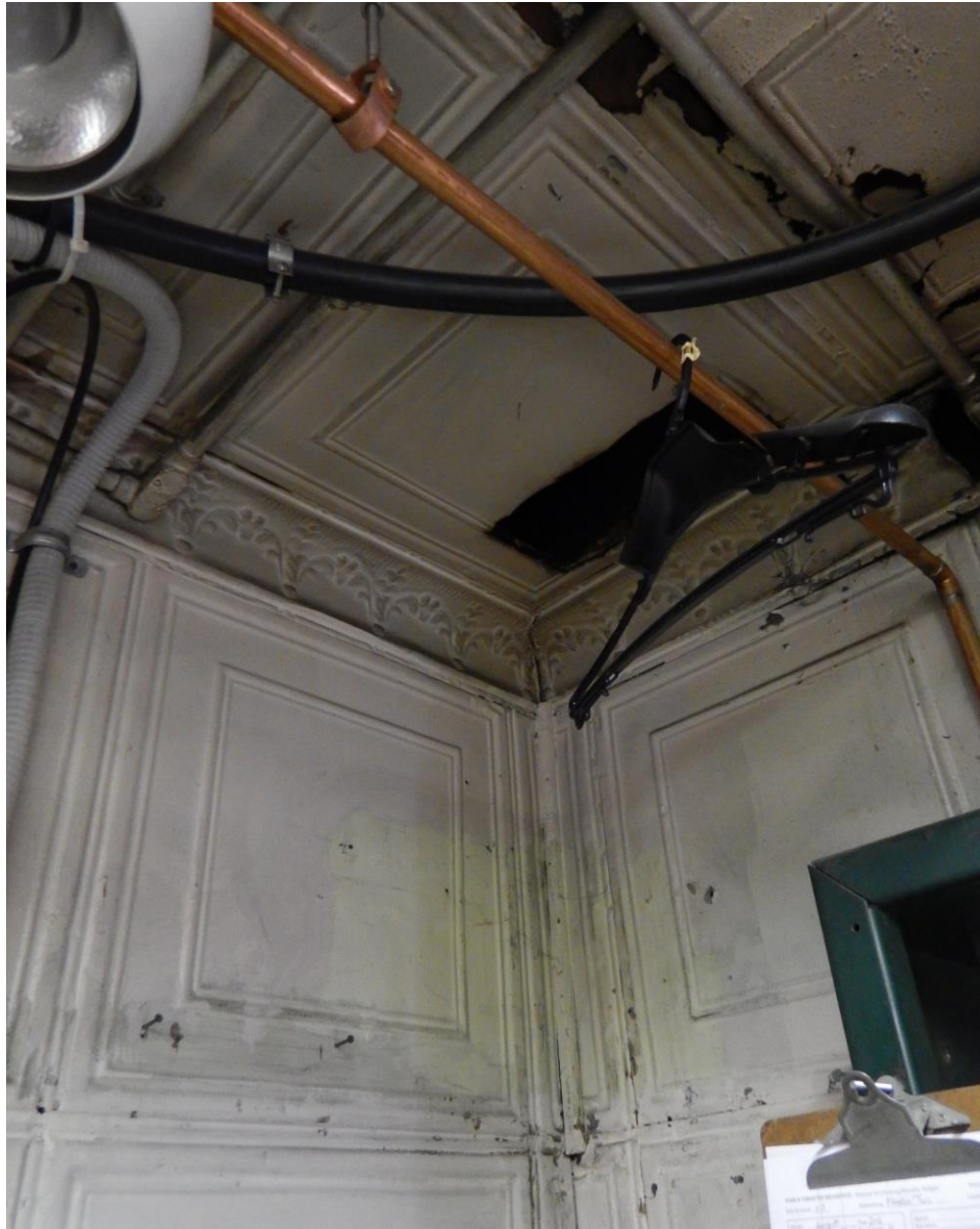
PHOTO 76. FIRST FLOOR TIN WALL AND CEILING DETAIL
