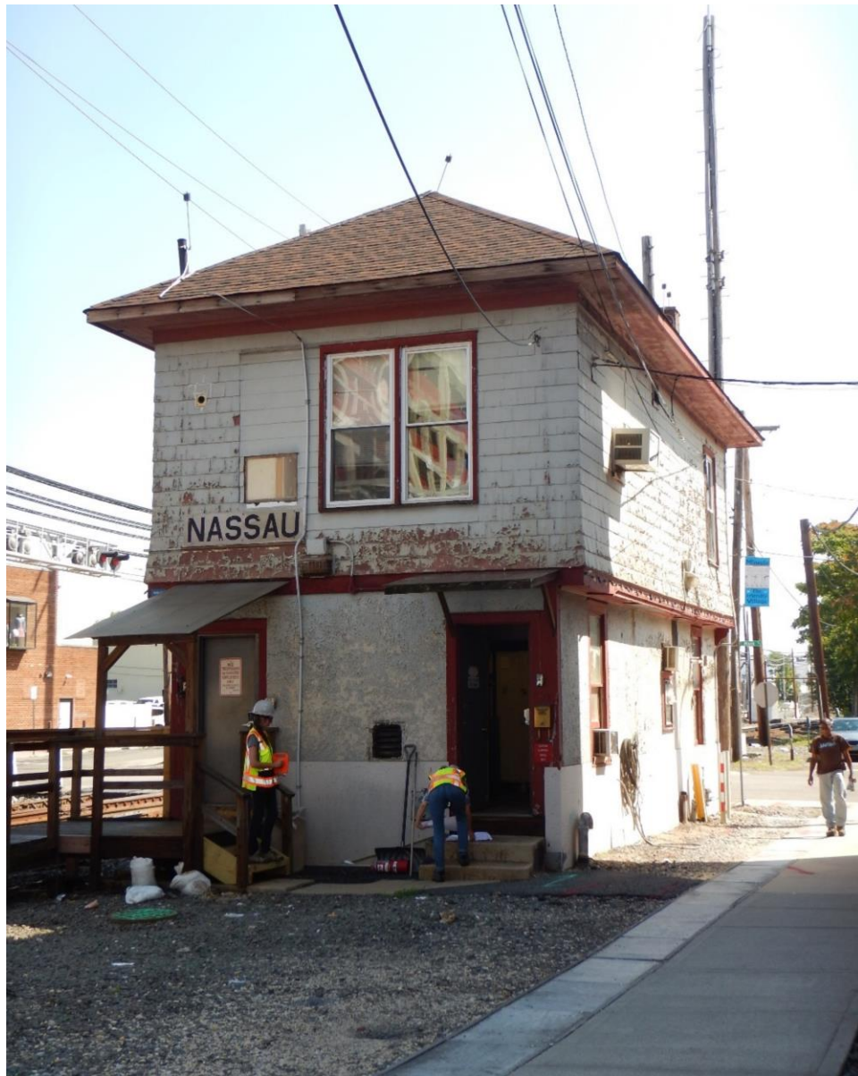
PHOTO 61. SOUTH AND WEST ELEVATIONS OVERALL
