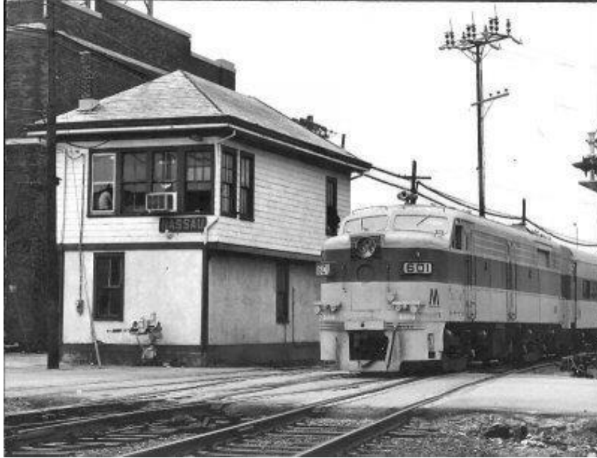
Fig. 15. East and north facades of Nassau Tower in May 1971, view looking southwest. The original fenestration pattern and multi-lite windows are still intact. Source: "LIRR Interlocking Towers & Cabins," http://www.trainsarefun.com/lirr/lirr%20towers/lirrtowers.htm , image courtesy of Richard Glueck.
