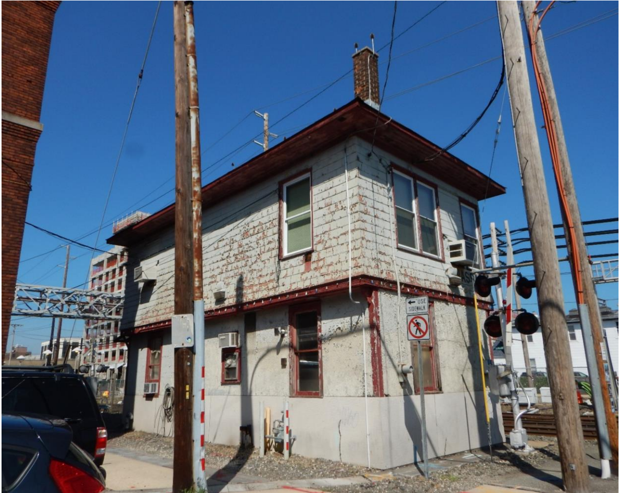
PHOTO 56. SOUTH AND EAST ELEVATIONS OVERALL
