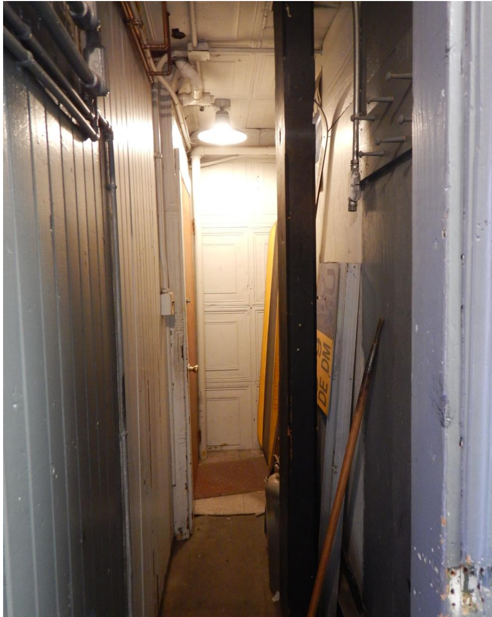
PHOTO 65. FIRST FLOOR ENTRY HALL FACING NORTH
