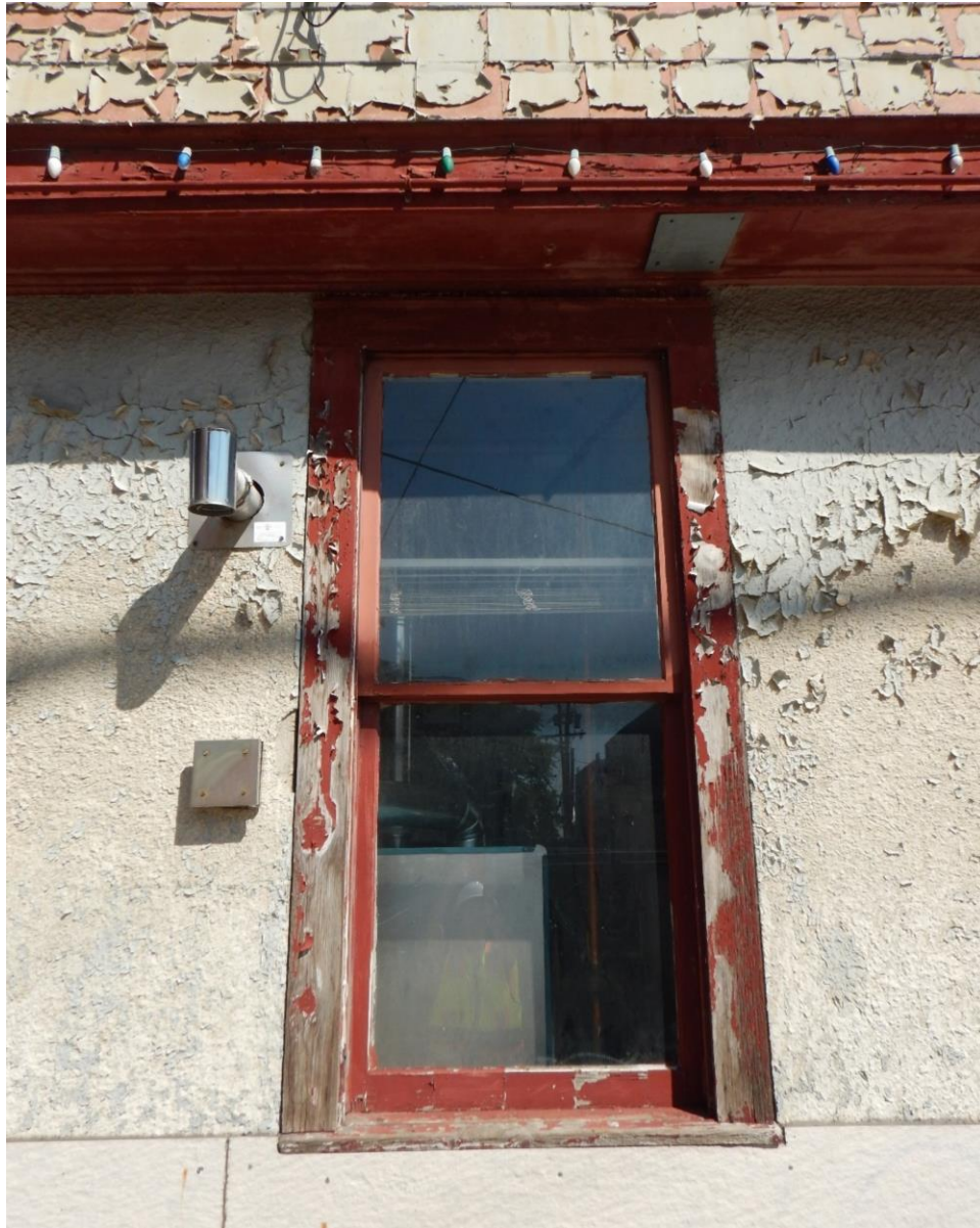
PHOTO 59. SOUTH ELEVATION WINDOW DETAIL
