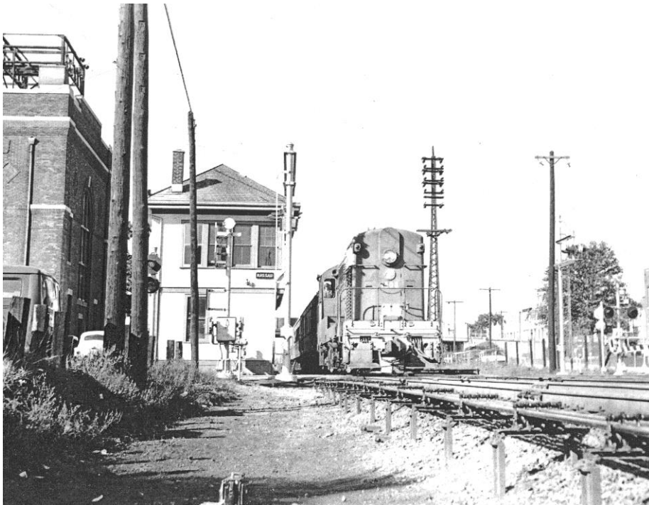
Fig. 14. The east facade of Nassau Tower c.1958, showing the four original window openings at the second story, view looking west. Source: Photographer: John Krause, image accessed from the Queens Public Library.
