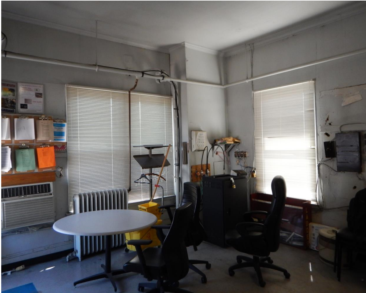
PHOTO 80. SECOND FLOOR FACING SOUTHEAST
