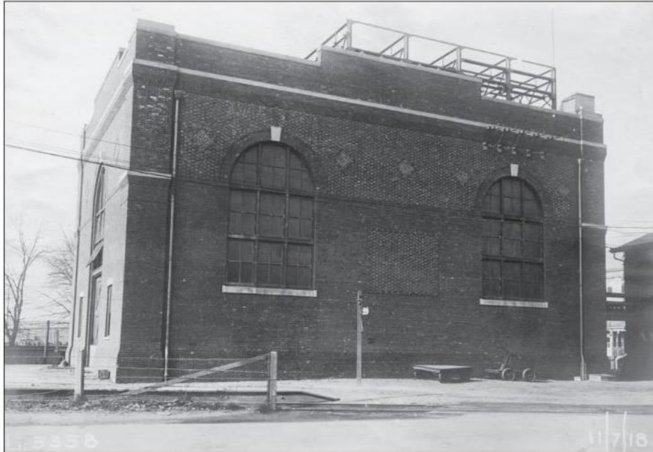
Fig. 7. The east and south facades of the Mineola Electrical Substation (substation No. 8) in a photograph dated November 7, 1918, eight years after the building's completion. View looking west from Main Street. The bridge between the substation and signal tower is still intact (visible at the far right). The garage addition has not yet been built. Little else had been altered between this photograph and the current appearance. Source: Long Island Rail Road: Oyster Bay Branch, 29 .
