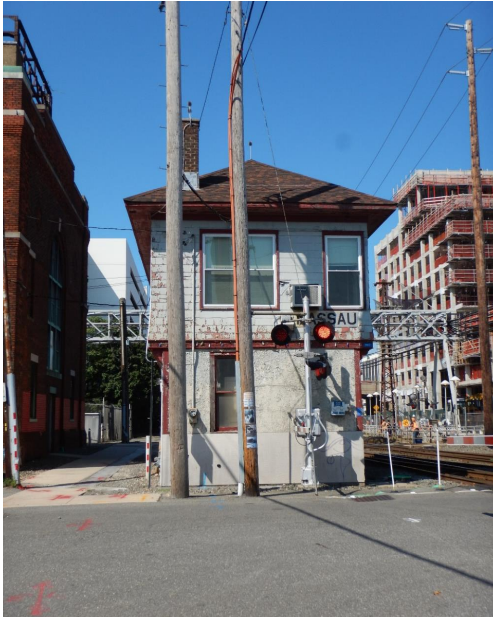
PHOTO 55. EAST ELEVATION OVERALL
