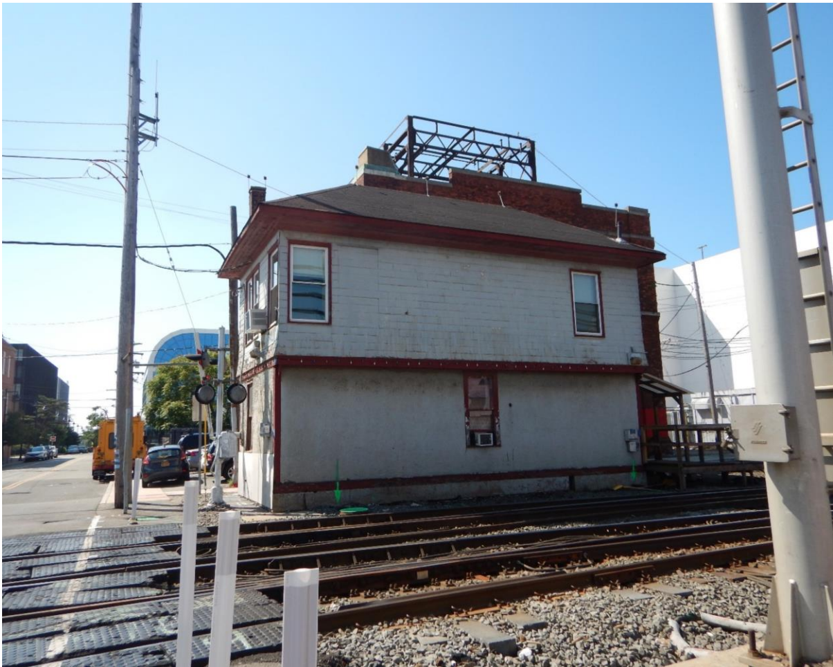
PHOTO 57. NORTH ELEVATION OVERALL
