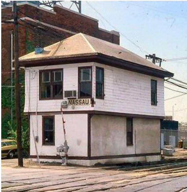
Fig. 16. Nassau Tower pictured in May 1979, view looking southwest. Windows at the north and east facades have been removed, openings infilled, and a new sign installed. Source: "LIRR Interlocking Towers & Cabins," http://www.trainsarefun.com/lirr/lirr%20towers/lirrtowers.htm , image courtesy of Steve Rothaug.
