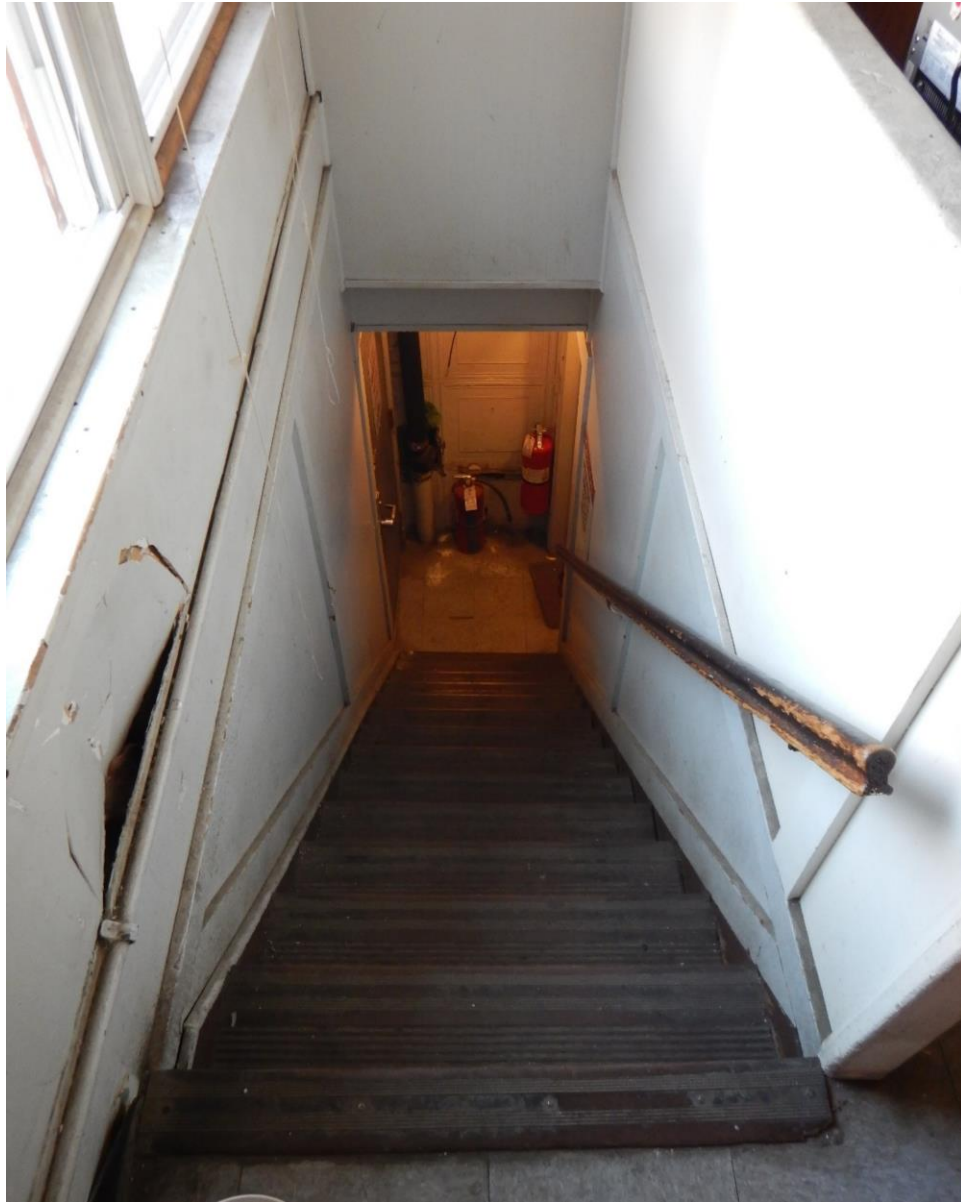
PHOTO 77. STAIRCASE TO SECOND FLOOR FACING NORTH
