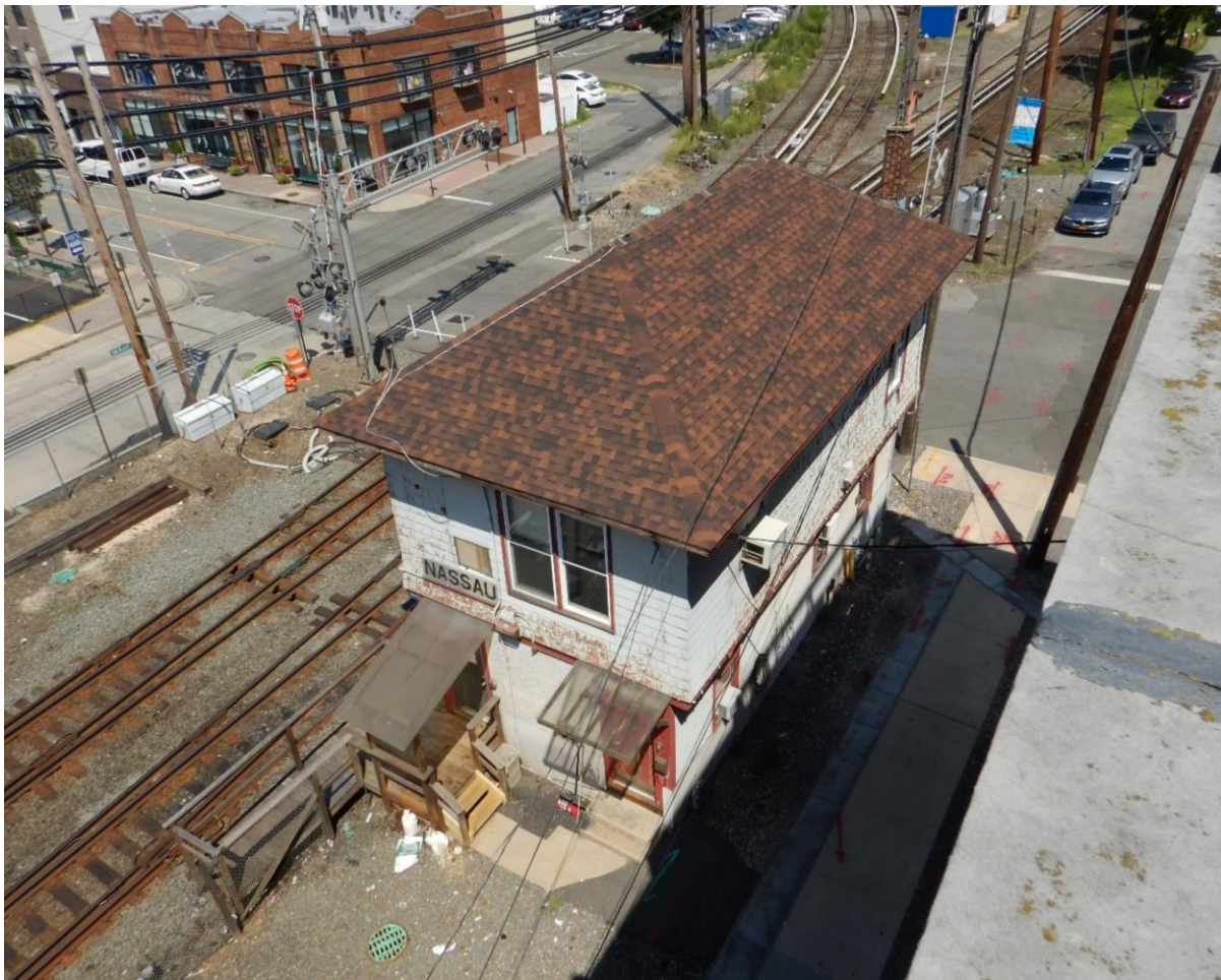
PHOTO 64. ROOF FACING NORTHEAST
