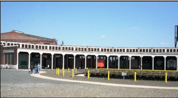
(Left) A portion of the roundhouse; it is intended to display the streamlined equipment around this turntable.
