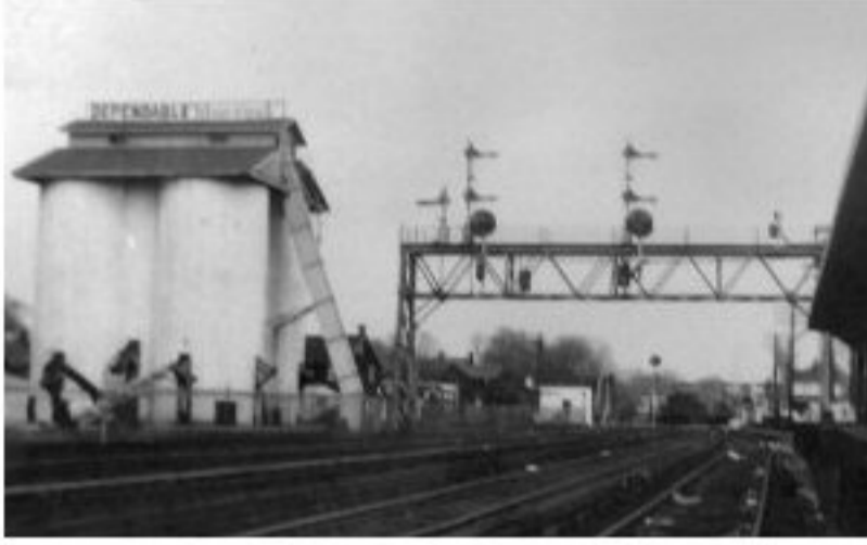
Babylon -Semaphores & replacement PRR Position Lights Dependable Fuel Co. Coal silos View E 1952 (Emery-SUNY)
