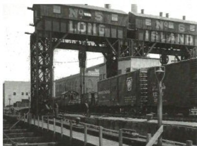
ALCO working bridges #5 and #6 Long Island City c. 1958 Photo/Archive: Ron Ziel
