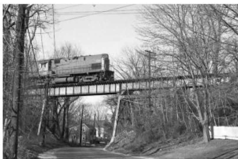
Old Town Rd., Setauket trestle C420 #202 eastbound - 12/1971 Photo/Archive: Dave Keller
