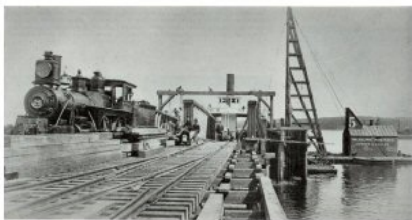
Oyster Bay float bridge 1892-1893 Archive: LIRR - LI Railroader
