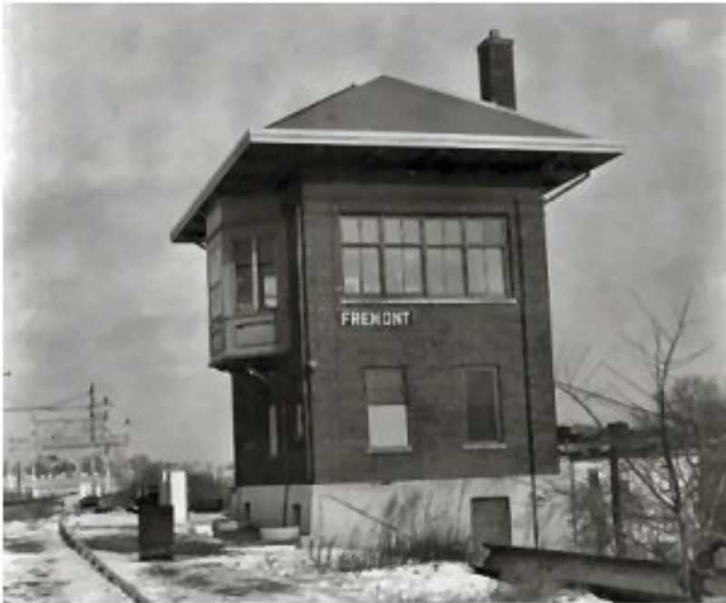
Abandoned Fremont Tower: 12/1970 Archive: Dave Keller
