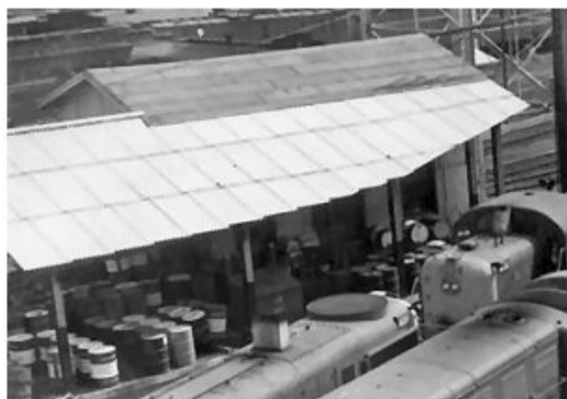
Oil House c.1962 Photo: LIRR Archive: Jim Gillin
