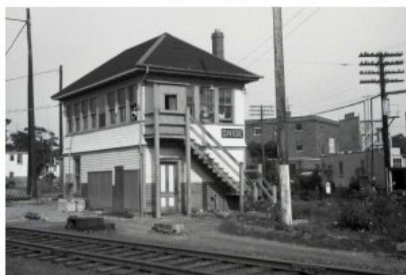
DIVIDE Tower, Hicksville View SE 1962 - Archive: Dave Keller
