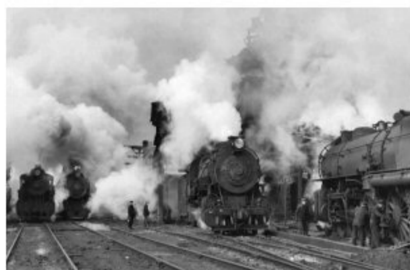
H10s #111 coal dock View W Morris Park engine terminal From left: G53, G5s and K2s Photo/Archive: LIRR c.1942
