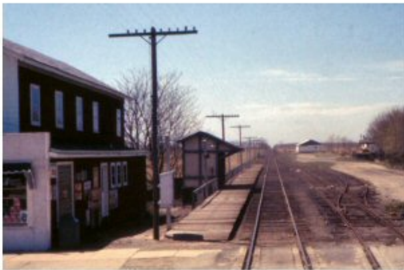
Peconic Shelter Shed 5/03/1964 view W Photo/Archive: Richard Makse
